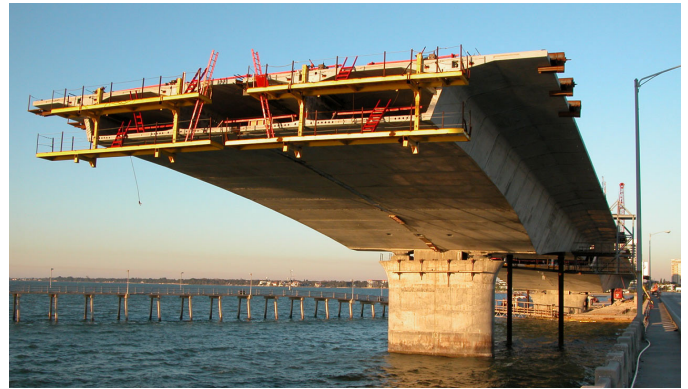
Two 9-foot diameter drilled shafts at each pier support the John Ringling Causeway bridge in Sarasota, Fla.
