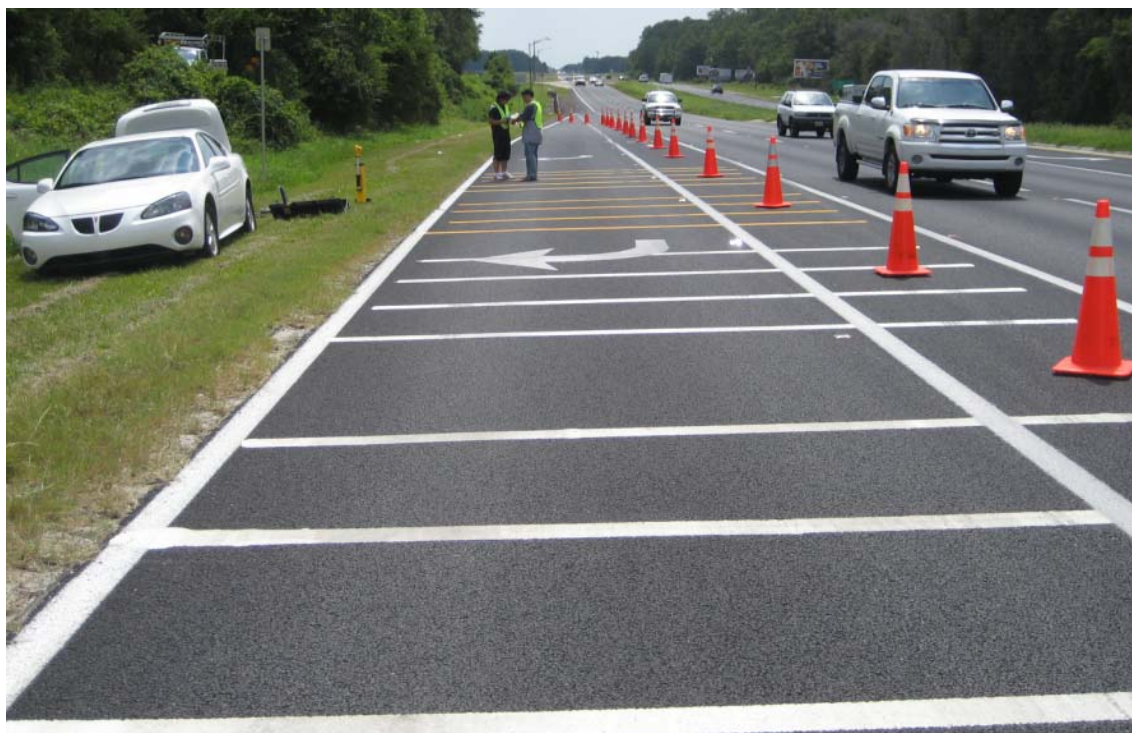
Figure 2-5. Test Site and Pavement Marking Configuration
