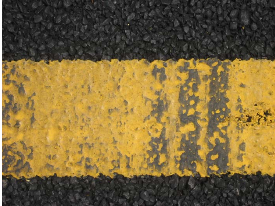
Figure 3-3. Wheel Tracking of Asphalt on to Surface of Pavement Marking (Product: C, Color: Yellow, Glass Beads: No)
