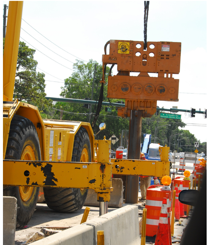
Complex work zones can be made safer with management tools.
