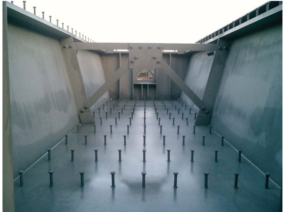
Double composite box girder
