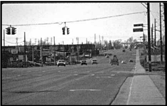
Figure 4: South Golden Road prior to reconstruction (5).
