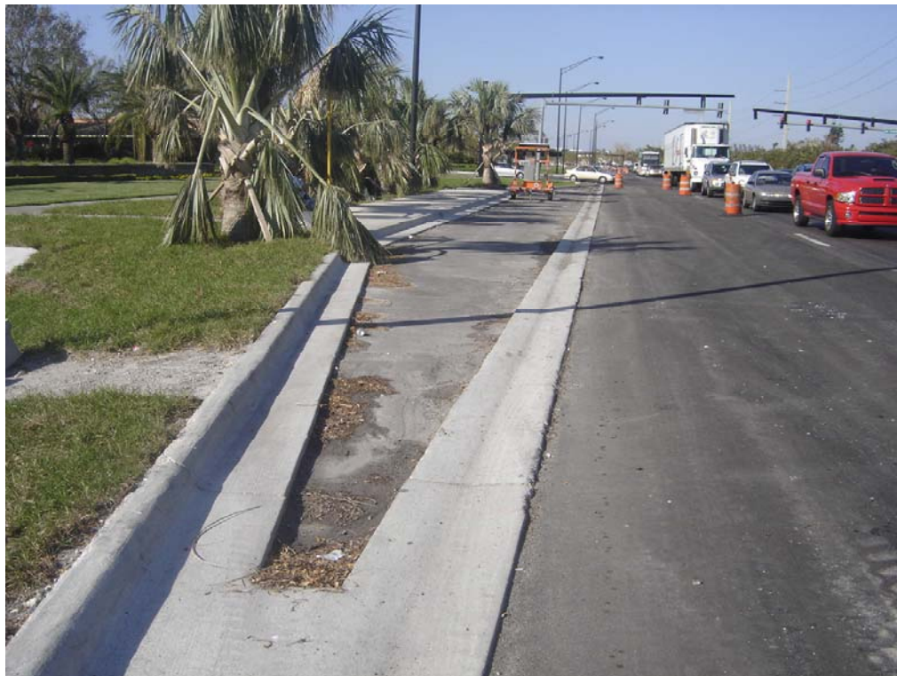
Figure 3.13. Pay Item No. 334-1-12 “SuperPave rebuild” GPS-measured on Nov. 10, 2005: Northbound View
