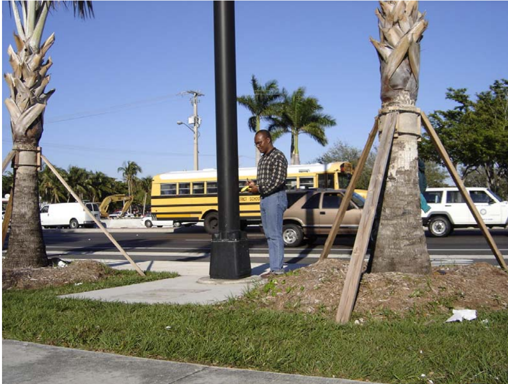
Figure 3.5 Light Pole and Part of Pay Item No. 522-1 “Sidewalk conc. 4in.” GPS-Measured on Feb. 11, 2005: Southbound View
