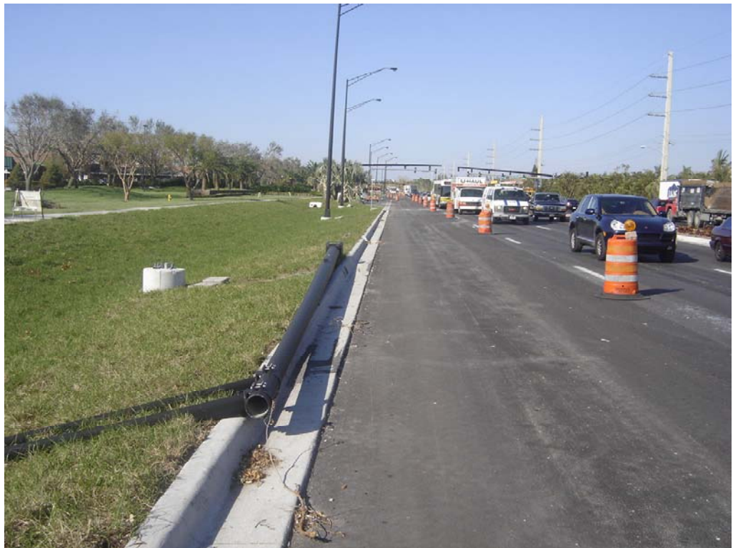
Figure 3.11 Northbound View of GPS-measured Pay items on Nov. 10, 2005:
