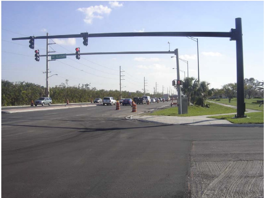
Figure 3.10 Southbound View of GPS-measured Pay items on Nov. 10, 2005:
