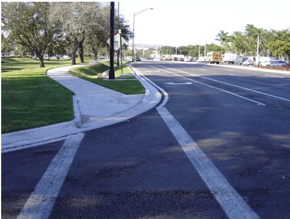
Figure 3.6. Pay Item No. 520-1-10 “Curb & Gutter Conc. Type F with Signs and Light Poles” GPS-Measured on Feb. 11, 2005: Northbound View
