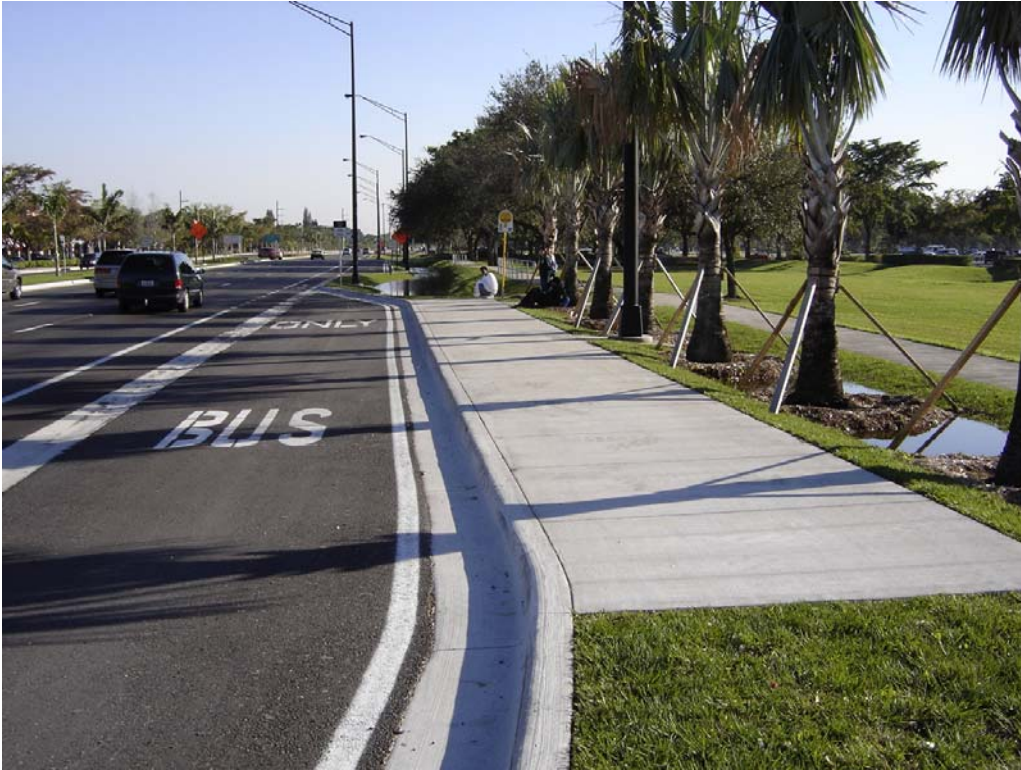
Figure 3.3 Pay Item No. 522-1 “Sidewalk 4in.” (Near Broward Mall) GPS-Measured on Feb. 11, 2005: Southbound View, Showing part of Pay items 520-1-10 “Curb & Gutter Conc. Type F”
