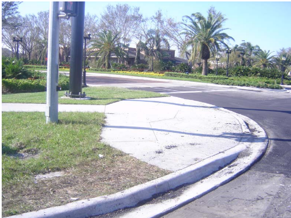
Figure 3.15 Pay Item No. 522-1 “Sidewalk Conc. 4 in.”” GPS-measured on Nov. 10, 2005: Northbound View
