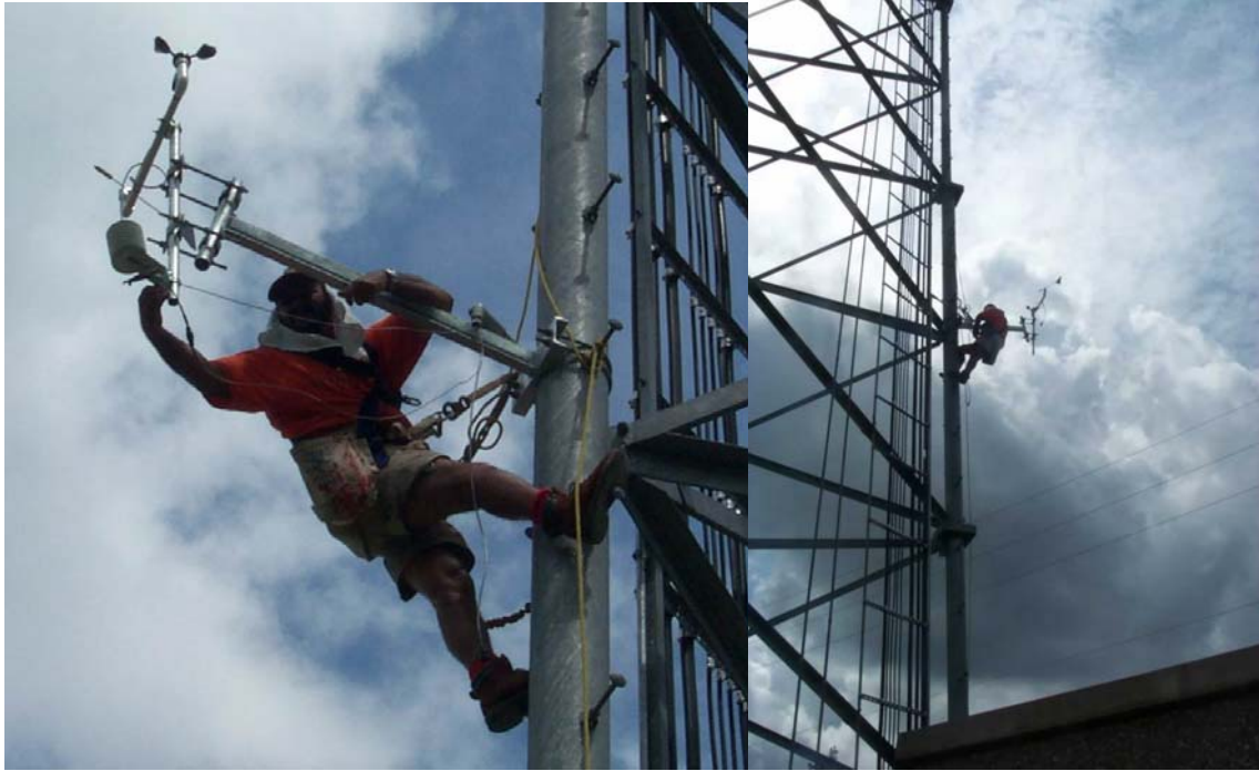
Figure 3: Installation of a 'basic weather station' on a tower in the RWIS Research Facility.
