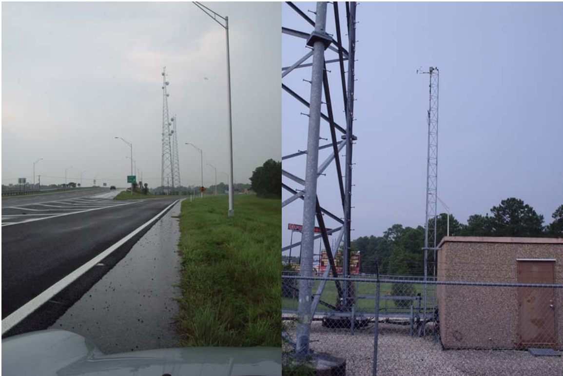
Figure 20: The “old” and “new” towers at “Gopher Ridge” (left picture), and the 30 foot tall tower installed beside the communications shelter for reinstallation of the weather sensors.
