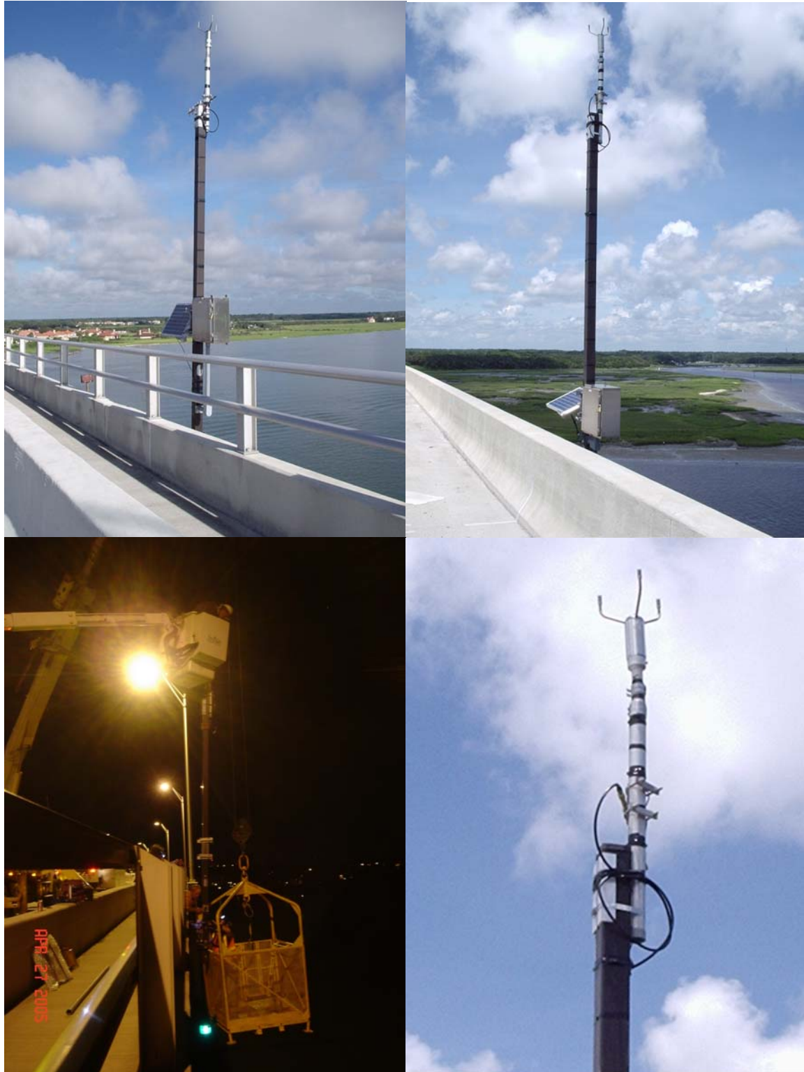
Figure 9: Completed installation of the wind sensors on the Vilano bridge (upper left) and the SR312 bridge (upper right). TCD, Inc. was contracted to provide installation services (lower left). Closeup of ultrasonic anemometer (lr).
