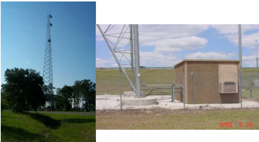
Figure 29: Photo on left illustrates how some MAS tower locations do not provide a desirable location for a weather station because of surrounding trees. Photo on right illustrates a more ideal location for a weather station.
