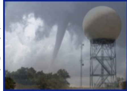
Figure 1. Nexrad Radar Radome [1]
