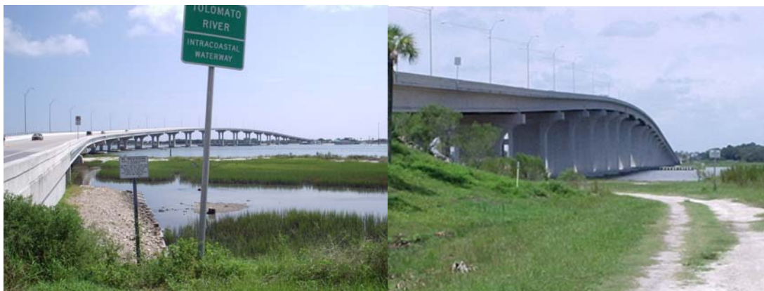
Figure 5: The two research facility bridge sites. Vilano Bridge (A1A) on the left, and SR312 bridge on the right.
