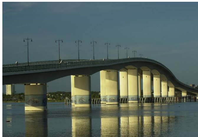
Figure 79. Broadway Replacement East Bound Bridge (BRB) General Span View.
