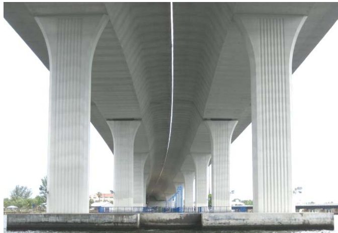
Figure 88. New Roosevelt (NRB) Substructure Elements.
