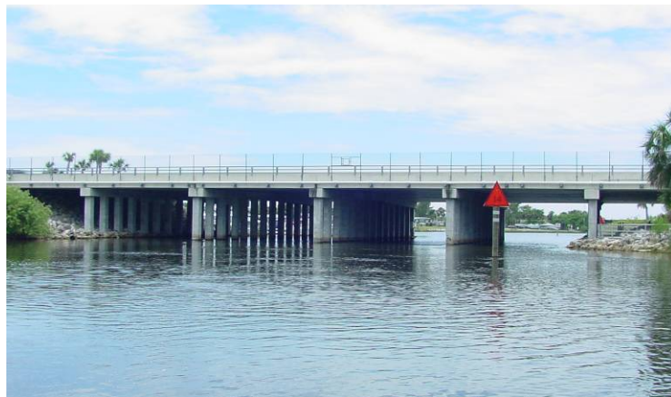
Figure 85. Turkey Creek Bridge (TCB) General Span View.
