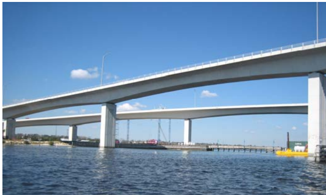
Figure 82. Seabreeze West Bound Bridge (SWB) Substructure Elements.
