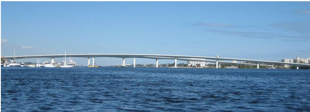
Figure 81. Seabreeze West Bound Bridge (SWB) General Span View.
