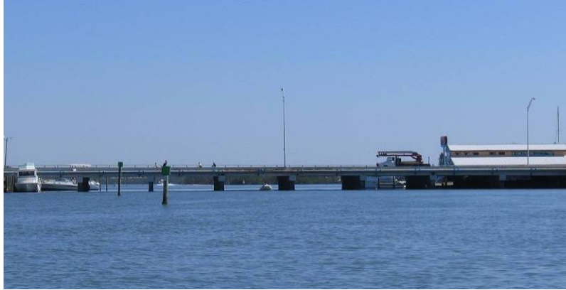
Figure 77. Hurricane Pass Bridge (HPB) General Span View.
