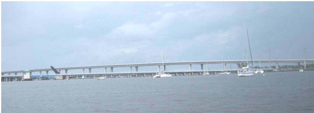
Figure 87. New Roosevelt (NRB) General Span View.
