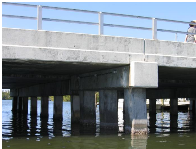
Figure 78. Hurricane Pass Bridge (HPB) Substructure Elements.
