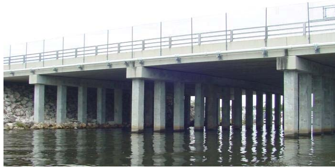
Figure 86. Turkey Creek Bridge (TCB) Substructure Elements.
