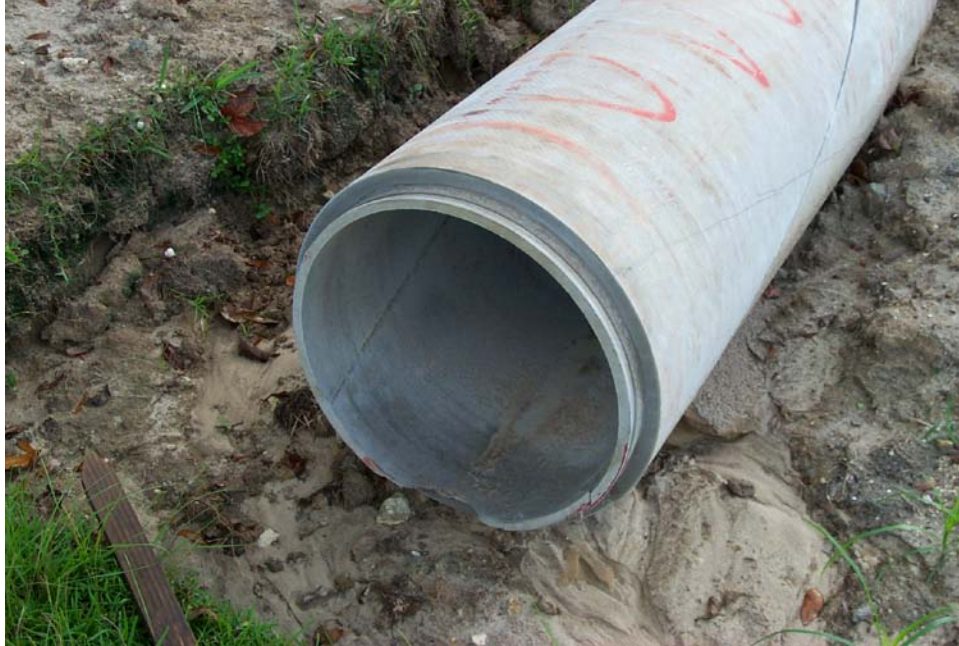
Figure A-3.5 Typical fiber reinforced concrete pipe.
