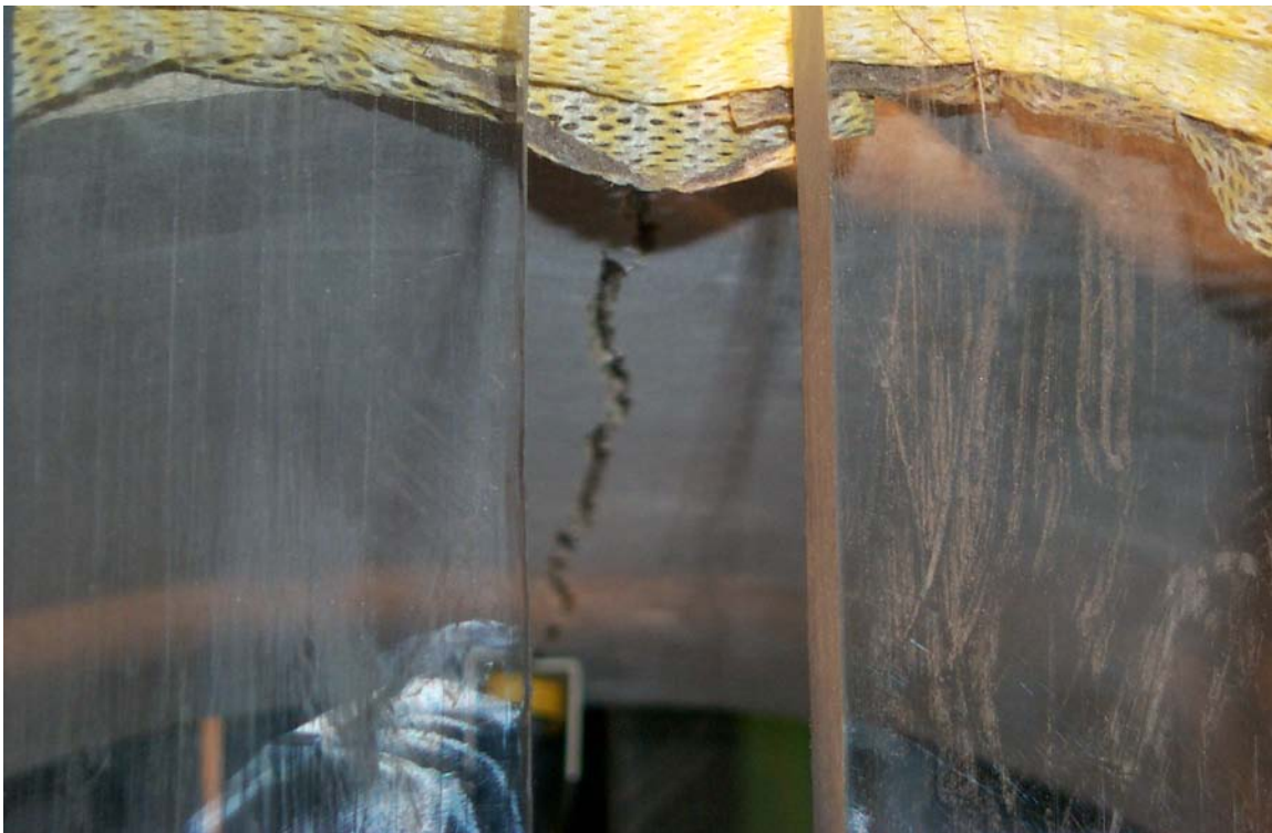
Figure A-2.10 Flexure crack at the crown of fiber reinforced concrete pipe.
