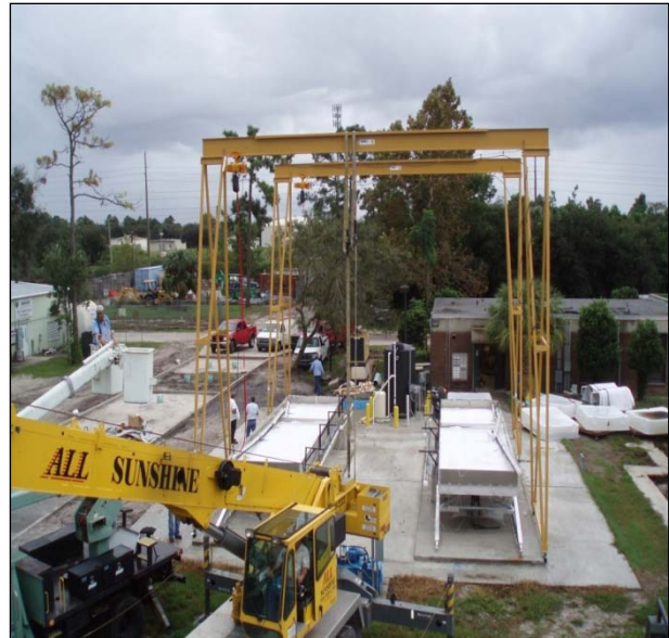
Figure 5 Installation of Gantry Crane System to Suspend Rainfall Simulator
