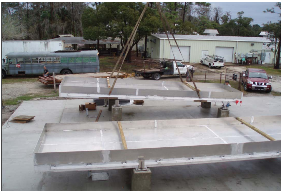
Figure 2 Installation of the Test Beds
