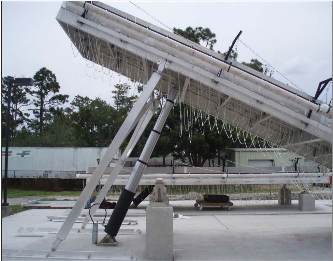
Figure 6 Safety Support Structure for the Test Beds
