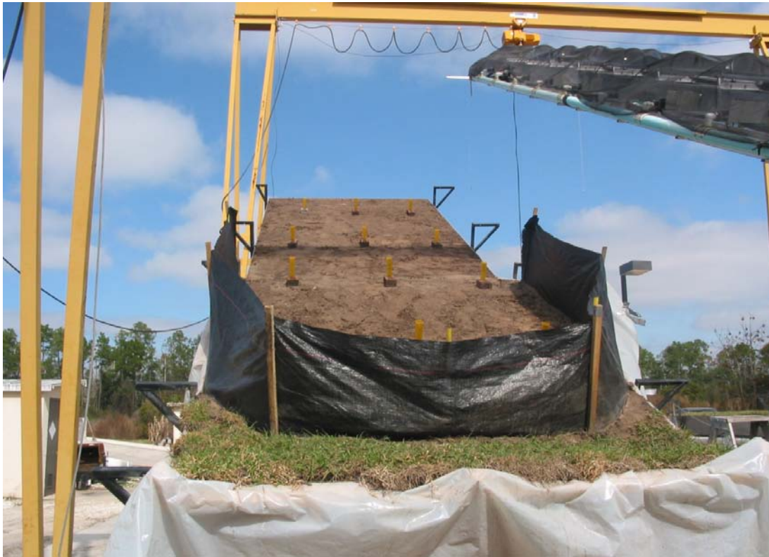
Figure 16 Silt Fence on the Test Bed before Evaluation with the Rainfall Simulator.
