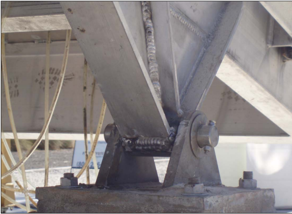
Figure 7 Additional Welding at the Pivot Points
