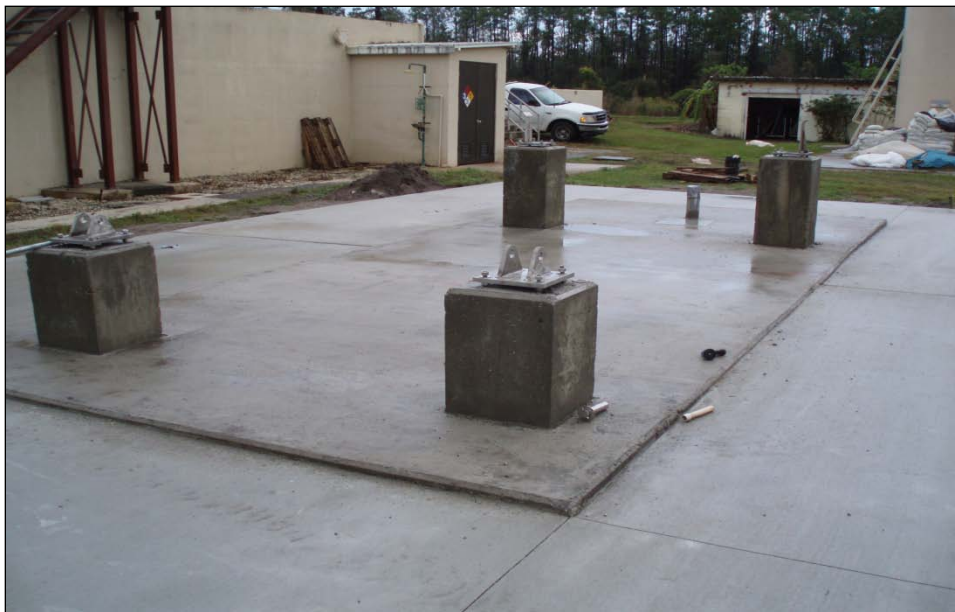
Figure 1 Foundation for One Test Bed
