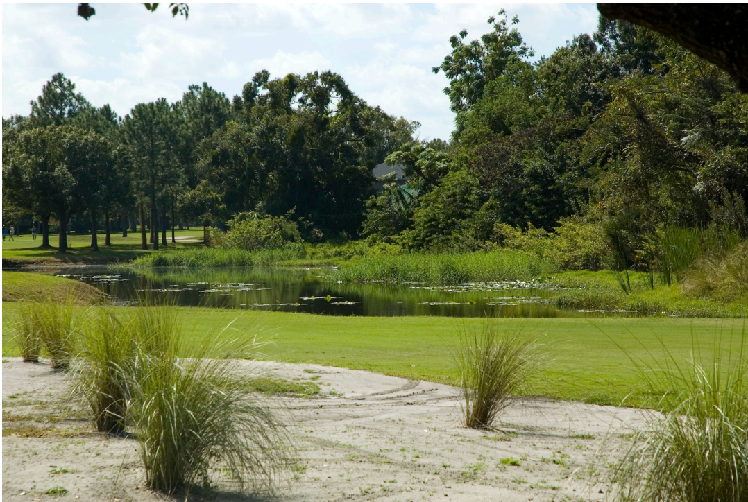
A golf course stormwater detention pond which filters runoff from nearby I-4 in Winter Park, Fla.
