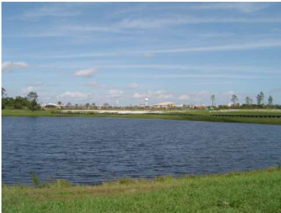
UCF South Irrigation Pond: View from south shoreline facing northeast.
