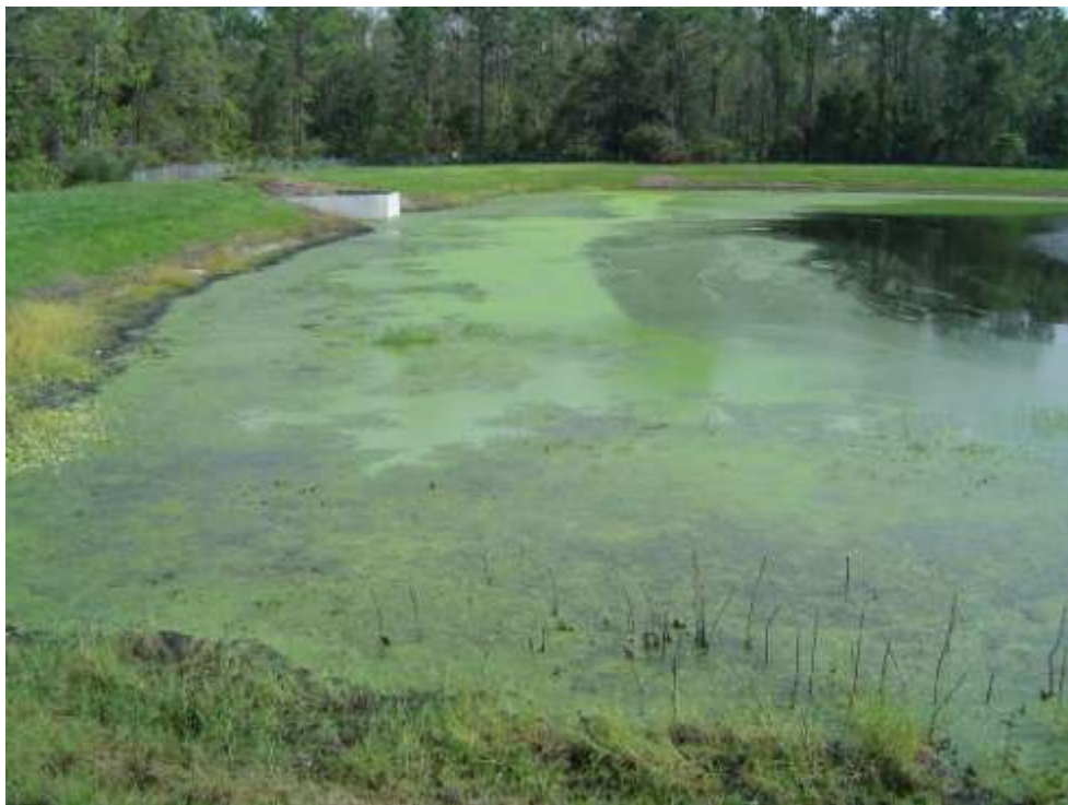
S.R. 417-5 Pond: View of algae along north shoreline.
