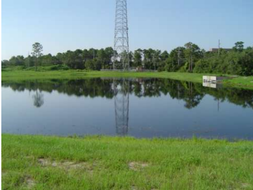
UCF South Irrigation Pond: View facing south from the north shore.
