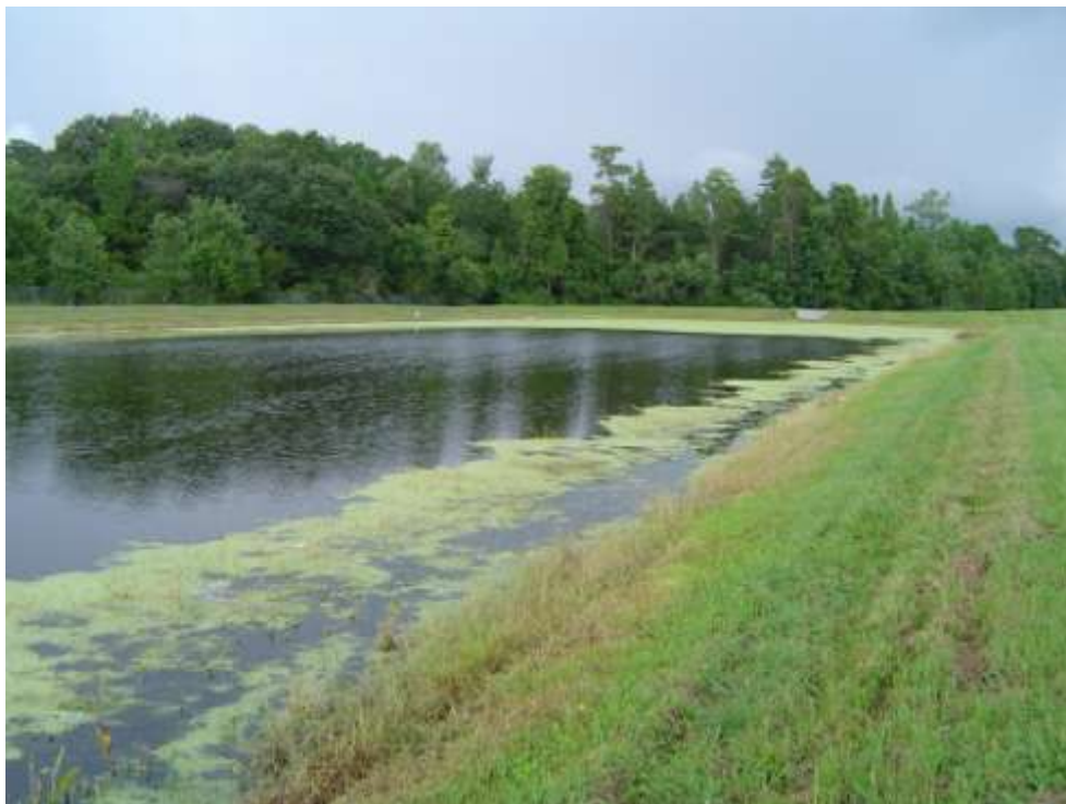
S.R. 417-2 Pond: View of east shoreline.
