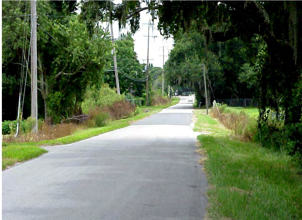
Pavement Repair Section at Glen Harwell Test Site
