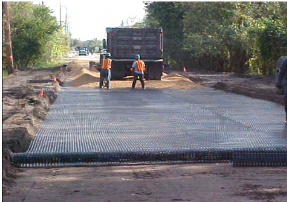
Beauchamp Road Test Site During Prior Repair Work
