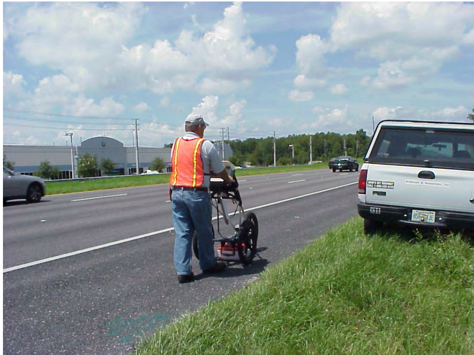
GPR Survey at Sandlake Road Test Site
