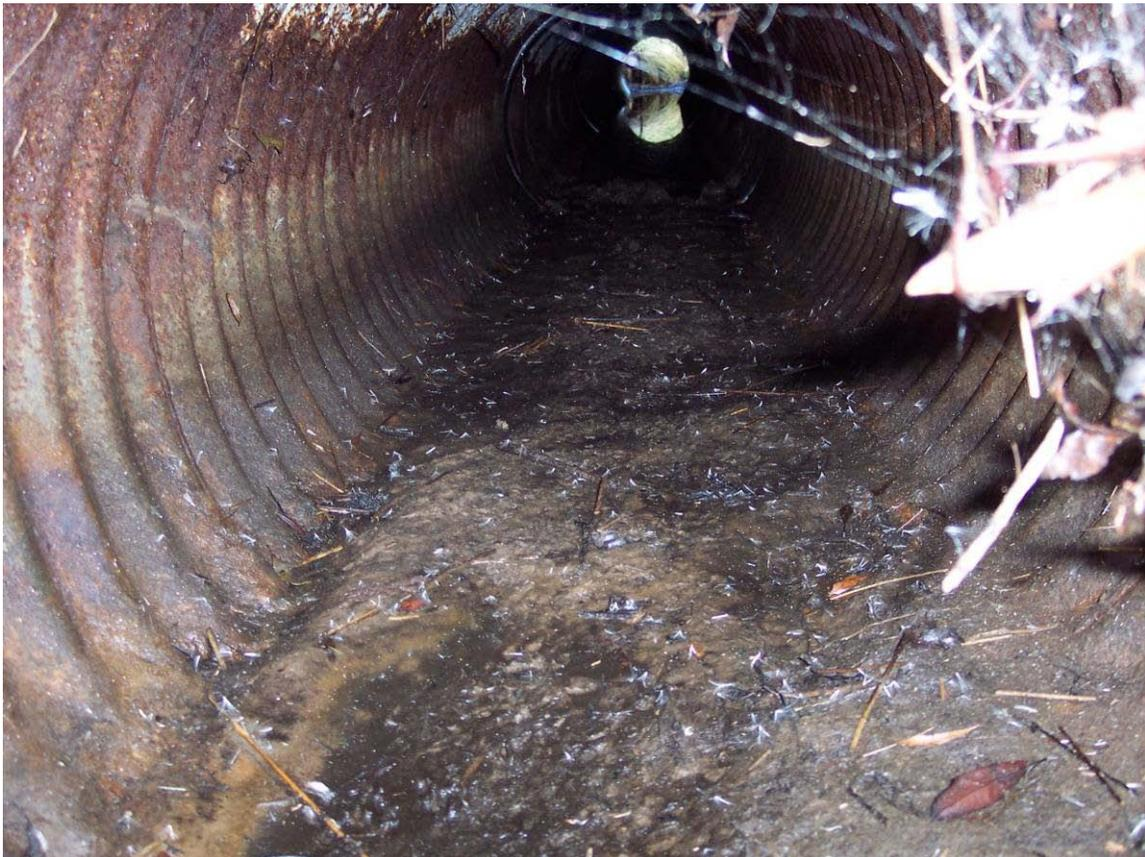
**Figure 10-2.** Corrosion is evident in an aluminized steel type 1 culvert pipe after 7 yr of service.
