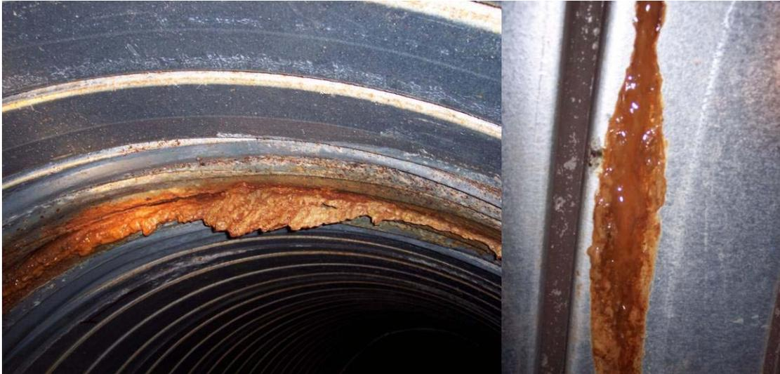
**Figure 10-1.** Possible bioslime oozing from damaged seam (left) and on inside wall (right) of in-service aluminized steel type 2 culvert piping.
