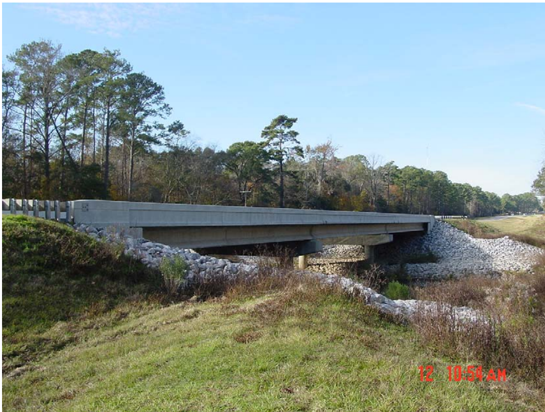
Figure 3.1. The tested bridge #500133 over Mosquito Creek.
