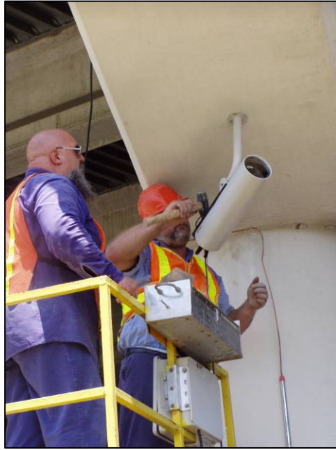
Figure 38: Camera Installation
