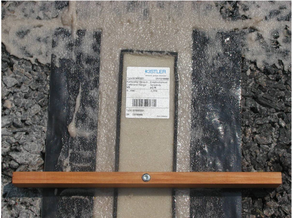
Figure 55: Installing Kistler strips on the road
