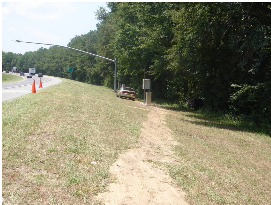
Figure 57: The site after equipment is installed
