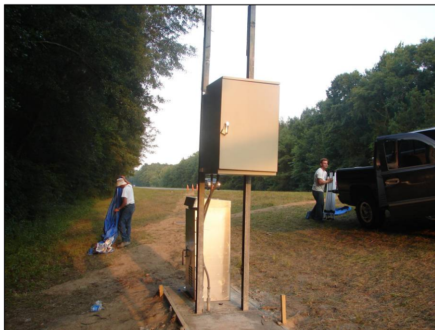
Figure 54: After installation completion
