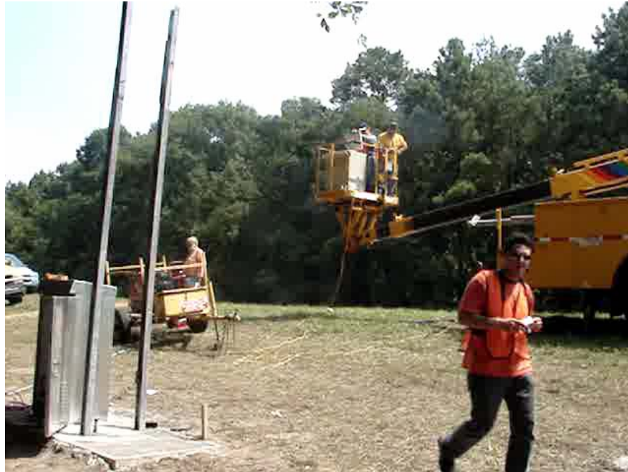
Figure 53: During onsite installation
