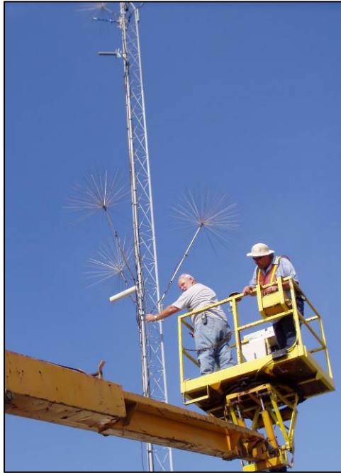
Figure 40: Antenna Installation at Flagler Weigh Station
