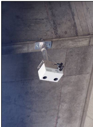
Figure 37: ASIM Sensor on the Middle of the Bridge.
