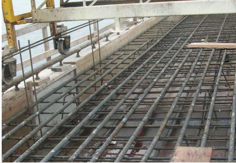
Figure B-1.3: Photograph of MMFX-II™ deck steel in place.
