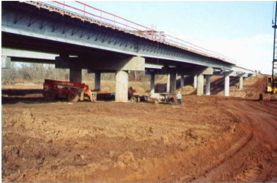
Figure F-1: General view of the I-35 northbound bridge.
