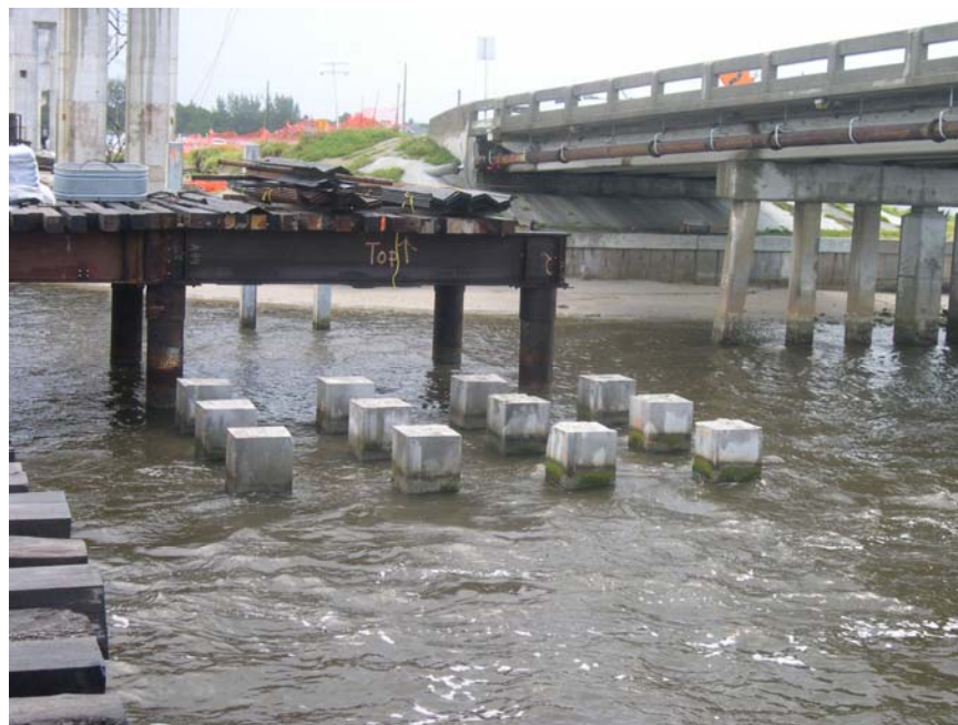
Figure B-2.2: Photograph of driven, cut-off prestressed piles for pier 11.
