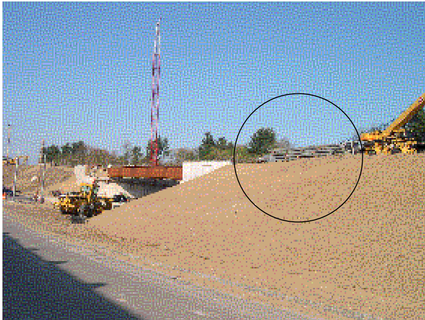
Figure E-1: General view of the Brown Avenue Bridge under construction.
