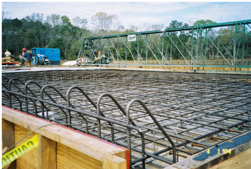
Figure G-3: View of 2205 stainless steel placement in Span 2.
