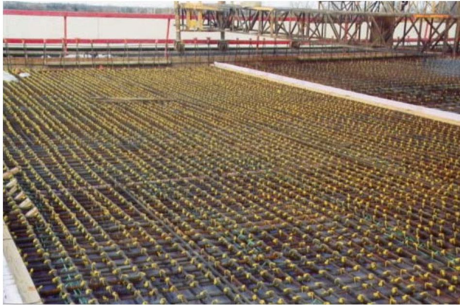
Figure F-2: Photograph of in-place deck reinforcing steel.
