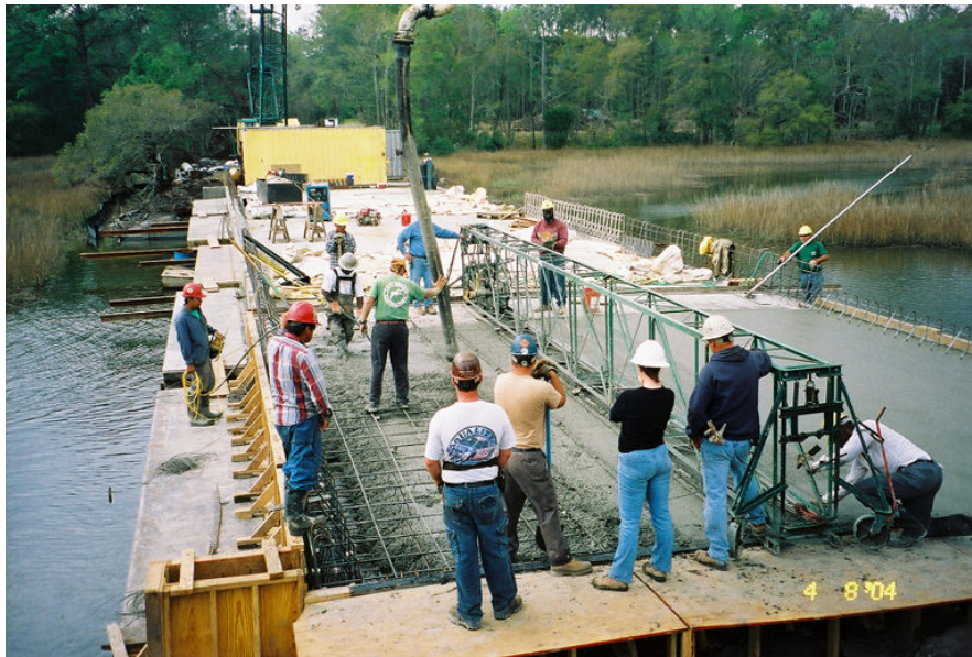
Figure G-1: General view of the bridge under construction.
