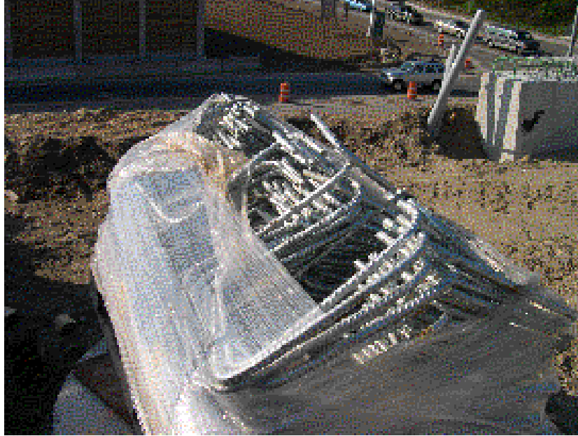
Figure E-7: Photograph of as-delivered galvanized bars at the Brown Avenue site after pulling back the plastic wrap.
