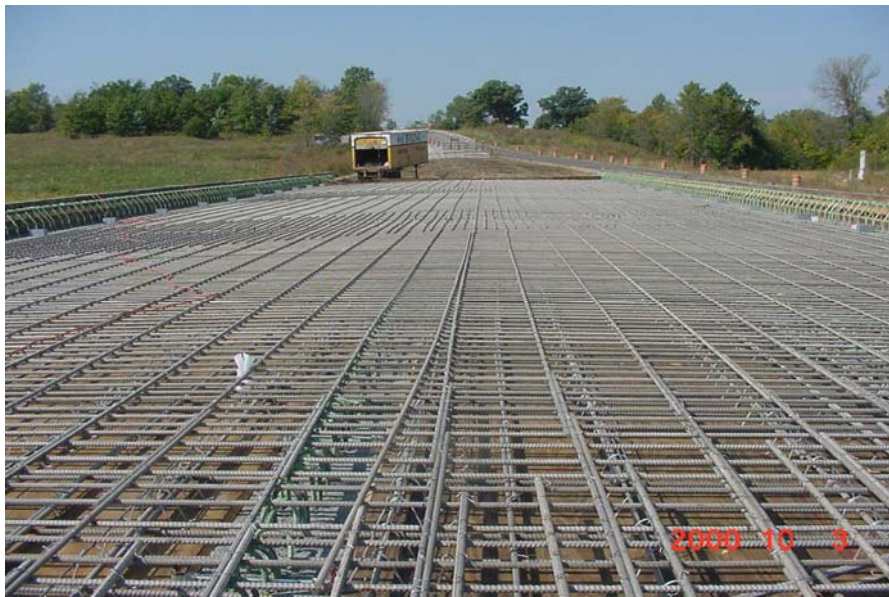
Figure C-3: Photograph of bridge deck with stainless steel in place.
