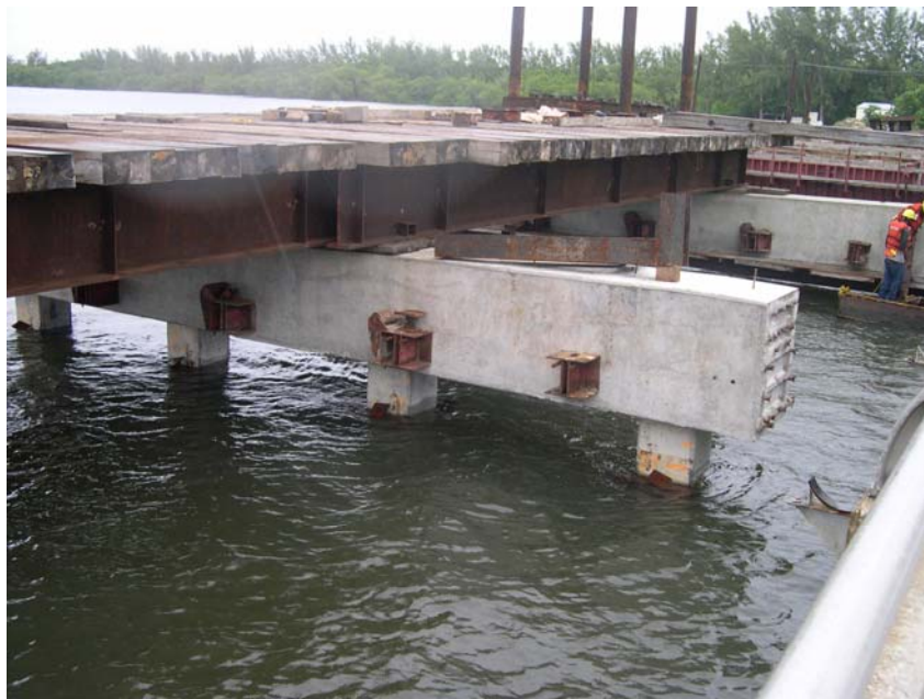
Figure B-1.2: Photograph of substructure components prior to decking.
