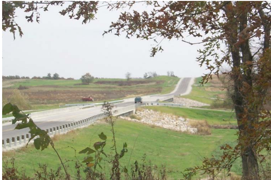
Figure C-1: General view of the Route 6 bridges.
