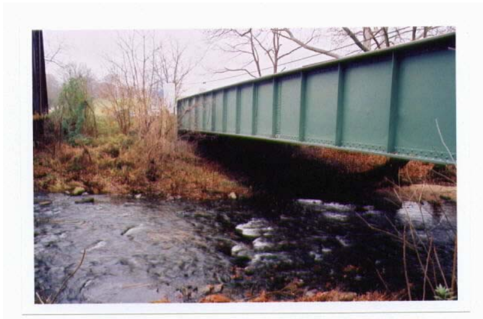
Figure A-1: Side view of Bridge No. 1-119.
