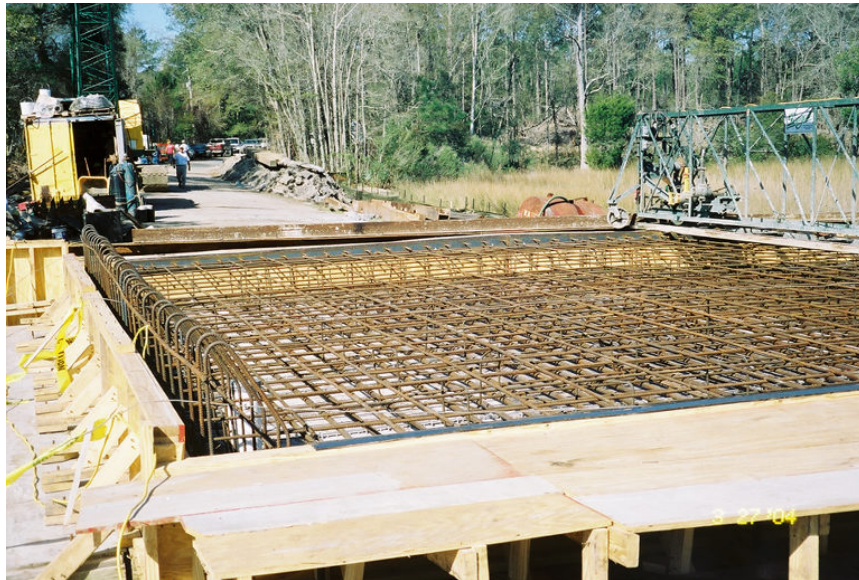
Figure G-2: View of MMFX-II™ placement in Span 5.
