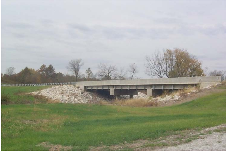
Figure C-2: Side view of Bridge Number 6059.
