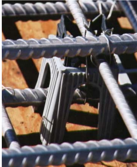
Figure D-8: Close-up view of a plastic chair to which bars are tied.
