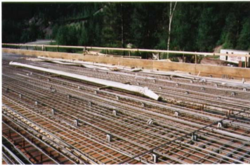
Figure D-7: Array of plastic chairs to which bars from both mats are tied.
