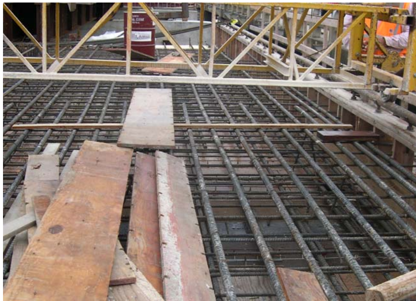
Figure B-1.4: Second view of MMFX-II™ deck steel in place.
