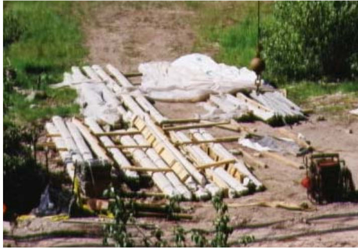
Figure D-2: Photograph of bundled/wrapped bars at the job site.
