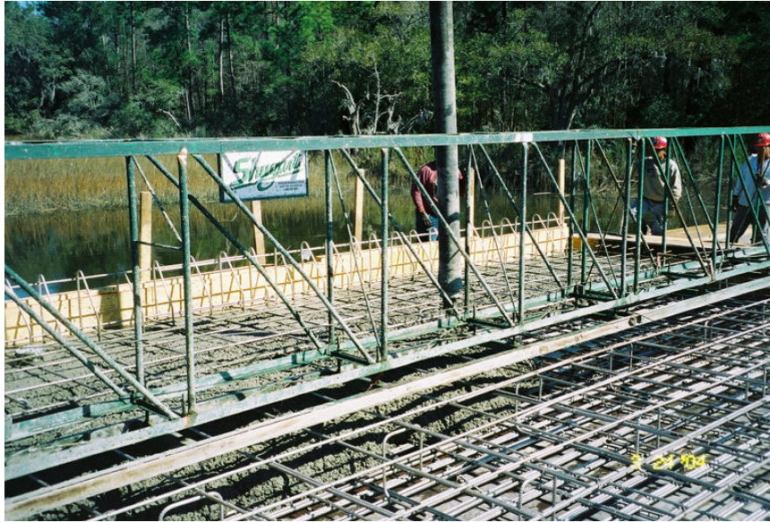
Figure G-4: View of in-place clad stainless in Span 3.
