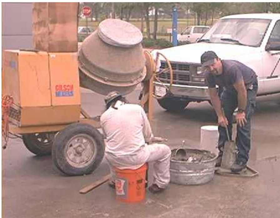
Figure 3.2: Concrete Casting & Slump Test
