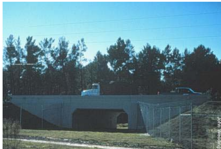
Underpass on SR-46 constructed at site of chronic bear-vehicle collisions. Underpass is a simple prefabricated concrete box 14.3 m long x 7.3 m wide x 2.4 m high. The dirt floor of the crossing is at ground level and the road was elevated over the structure to allow bears to easily see through the structure. Vegetation was planted to provide entrance and exit cover (Roof and Wooding 1996).
