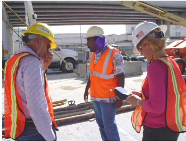
Figure 3.9: Data Recording from Sacrificial Sensors (IntelliRock™ System)
