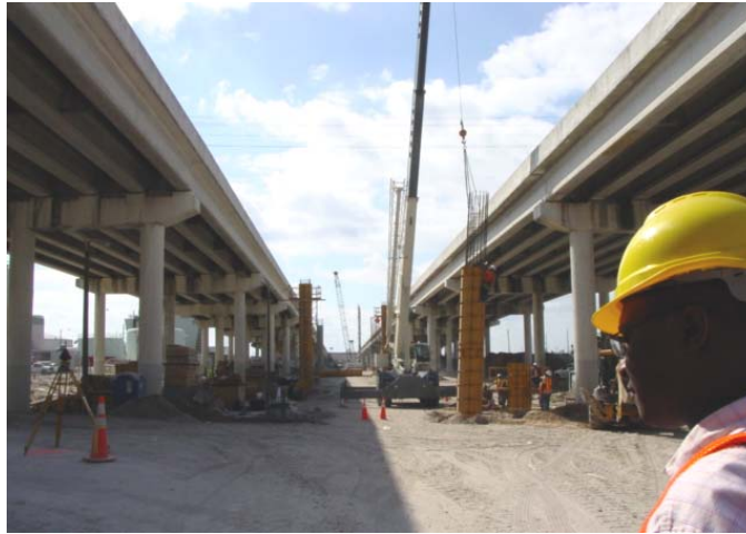
Figure 3.6a: A Longitudinal View of the Project
