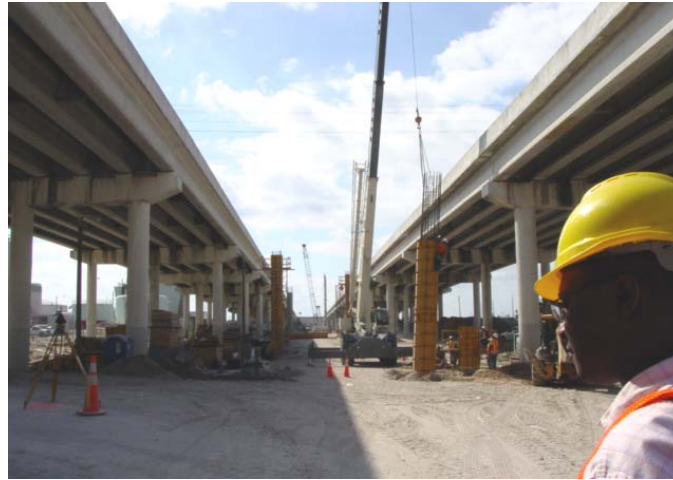
Figure 3.6a: A Longitudinal View of the Project
