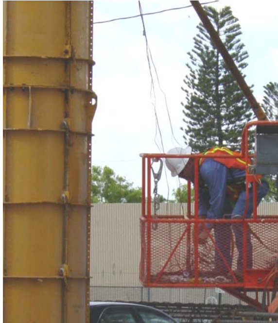
Figure 3.8c: Sensors Wires Coming Out from the Scaffolding of a Column
