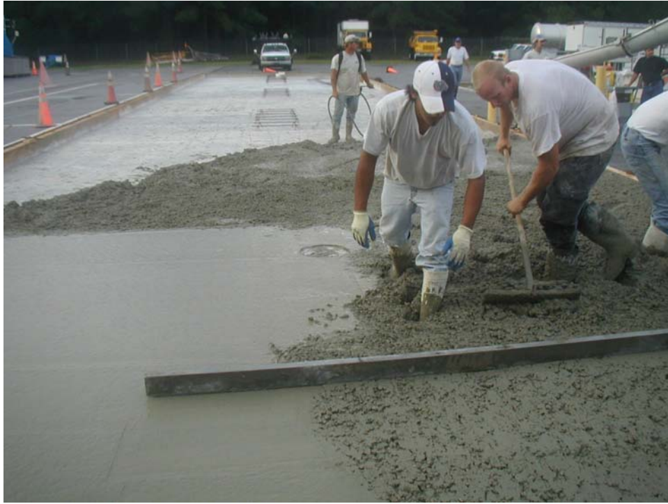
Figure 2. Placement of concrete on test track
