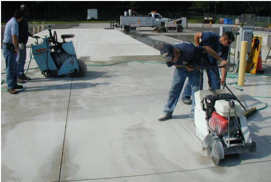
Figure 20. Cutting of a concrete slab (12 ft \times 16 ft) into small pieces (3 ft \times 4 ft)
