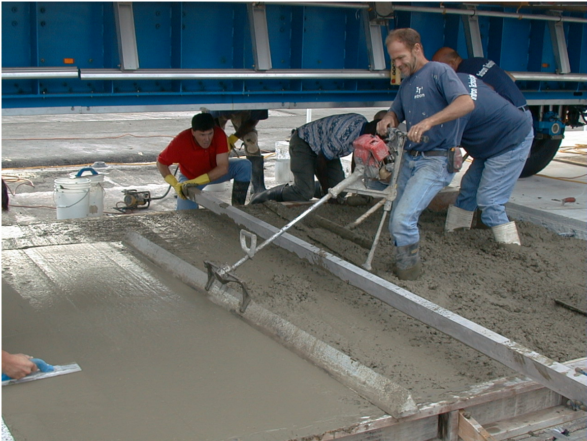
Figure 31. Leveling of concrete surface
