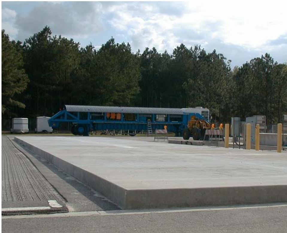
Figure 3. Finished concrete test track
