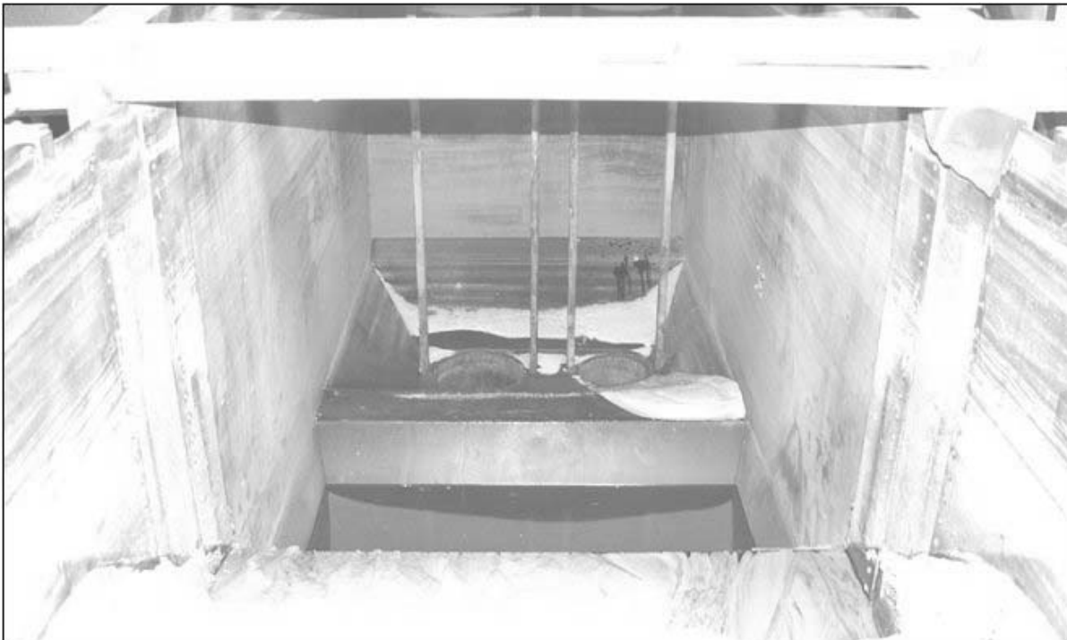
Figure 3.7 Catch basin at downstream end of flume.
