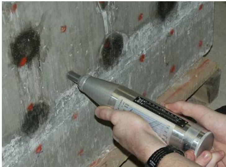
Figure 4.9: Rebound hammer testing.
