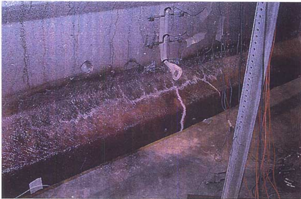
Figure 4-36: Test Specimen 5 at Failure Showing Rupture of FRP at Midspan
