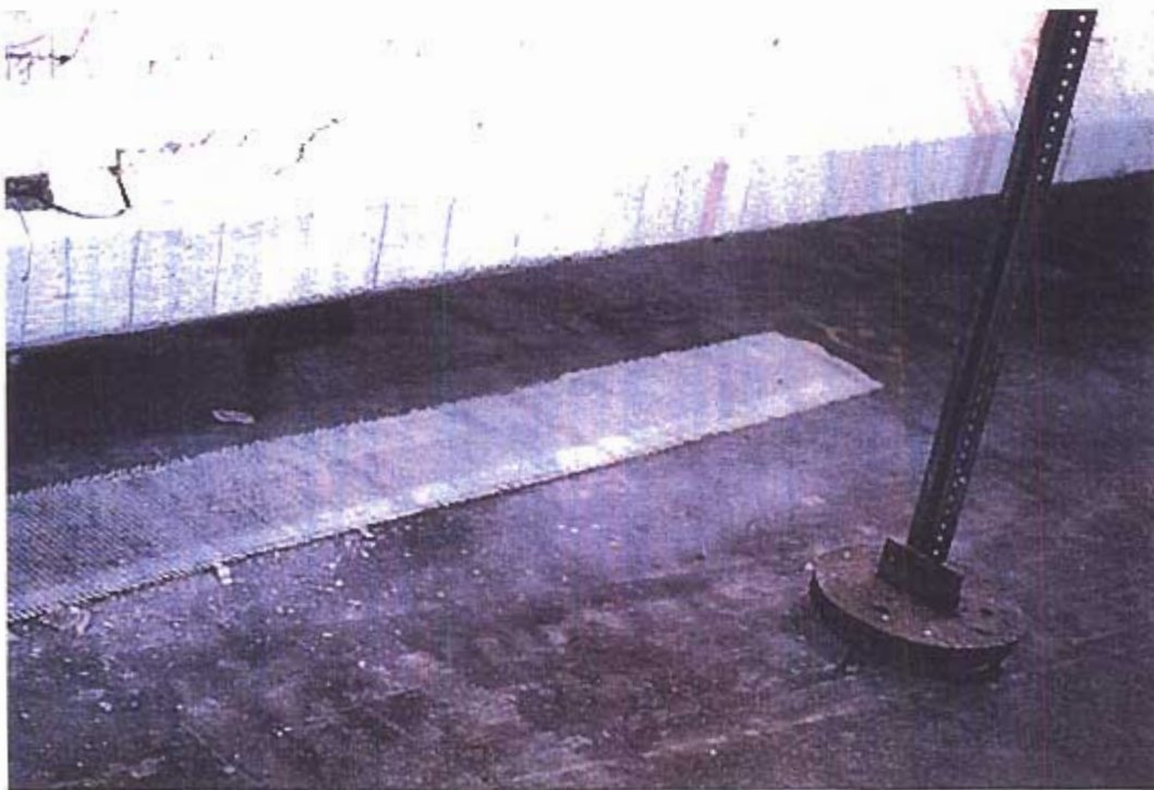
Figure 4-28: Test Specimen 4 at Failure Showing Separation of FRP
