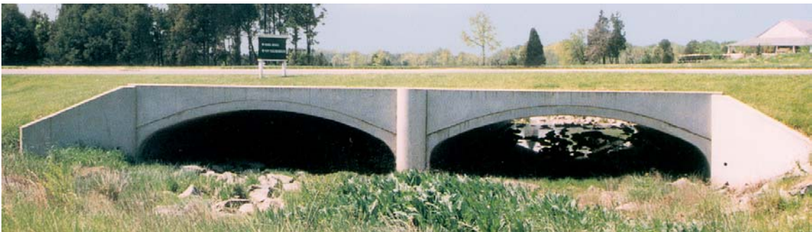
Figure 1.9: CON/SPAN Double Cell Precast Arch Culvert
