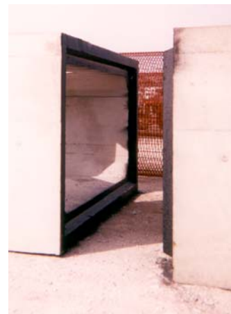
Figure 3.12: Tongue and Groove Joint
