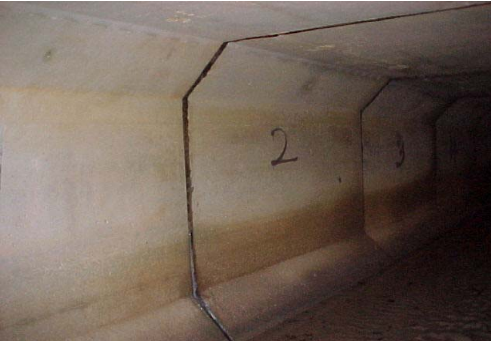
Figure 3.3: Interior View of Culvert Sections
