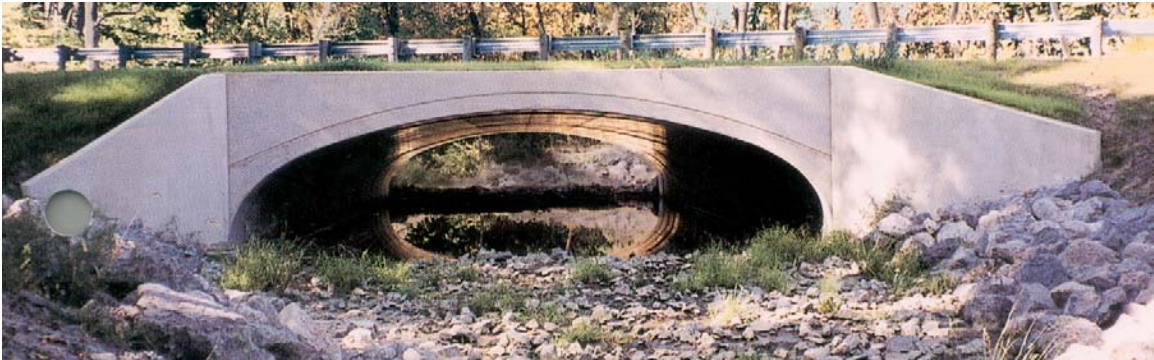
Figure 1.8: CON/SPAN Single Cell Precast Arch Culvert
