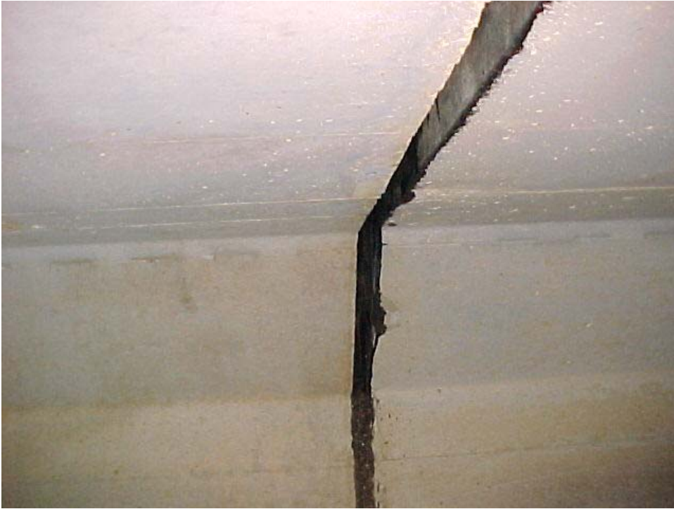
Figure 3.4: Joint Between Culvert Sections
