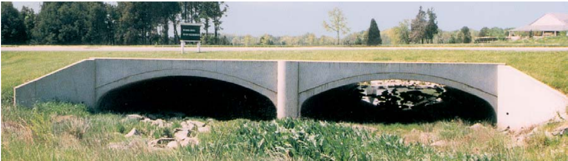
Figure 1.9: CON/SPAN Double Cell Precast Arch Culvert
