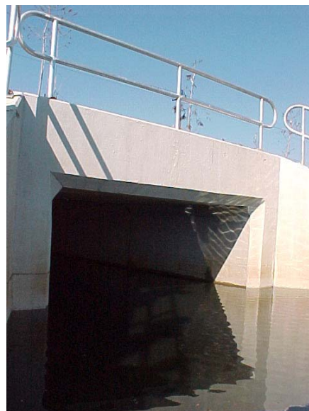
Figure 3.2: Exterior View of Culvert
