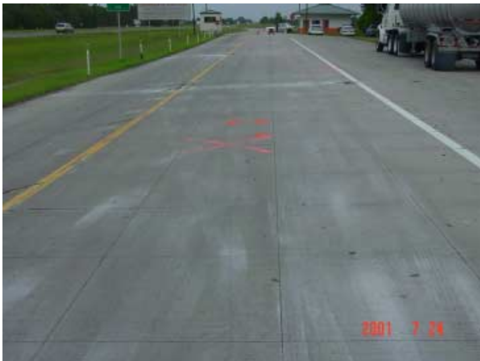
Figure 3.15 General View of Test Section S4E
