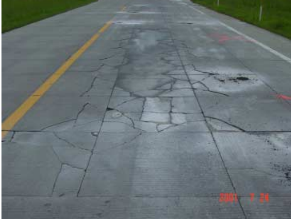
Figure 3.22 General View of Test Section S6E at the Beginning
