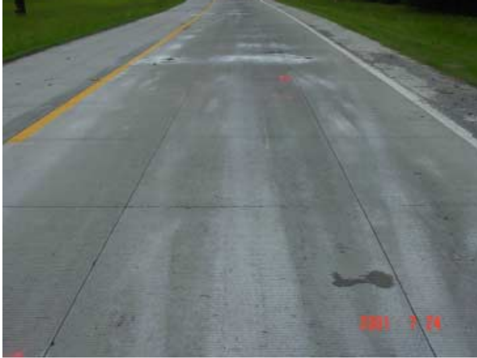
Figure 3.8 General View of Test Section S2W
