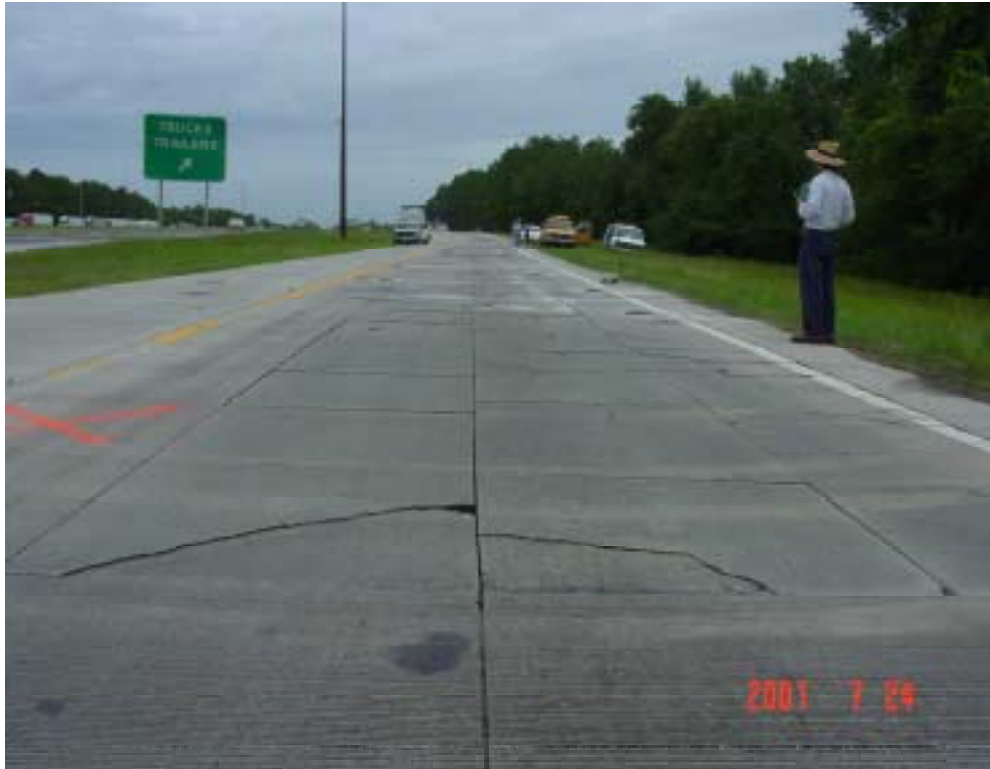
Figure 3.3 General View of Test Section S1W
