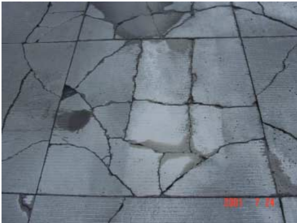
Figure 3.23 Shattered at the Beginning of Section S6E
