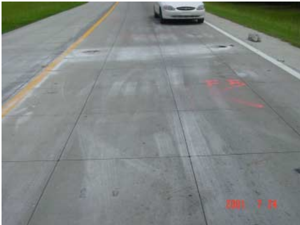
Figure 3.11 General View of Test Section S3W
