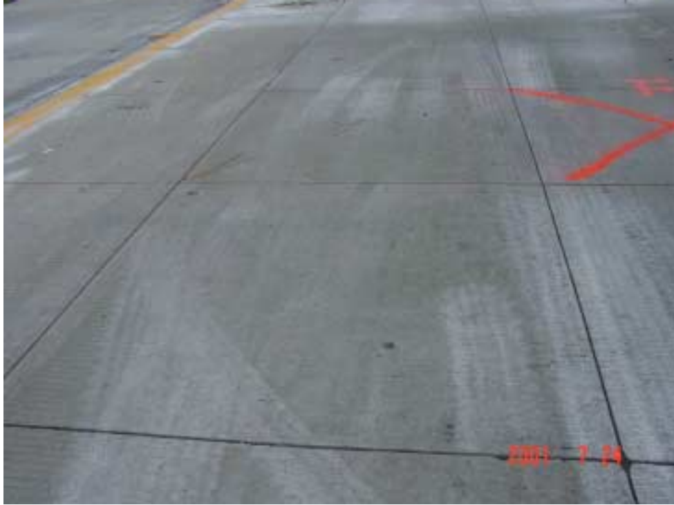
Figure 3.12 Close-up of Panels B15 and C15 of Test Section S3W
