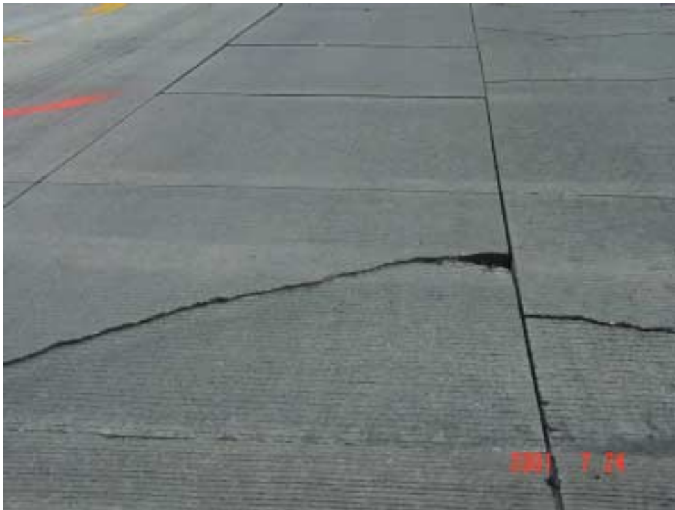
Figure 3.4 Close-up of Panels B2 and C2 of Test Section S1W
