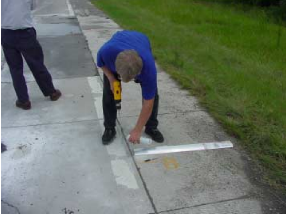
Figure 3.25 Drilling Holes for Thermocouple Installation
