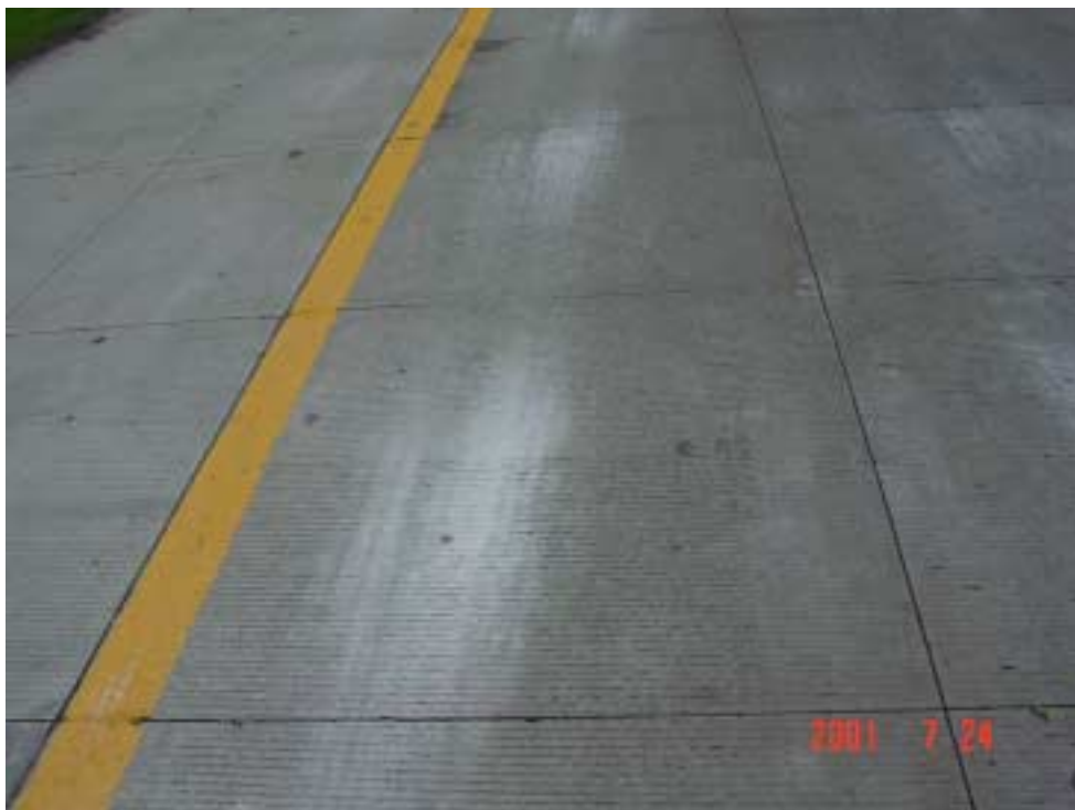
Figure 3.9 Close-up of Panel A22 of Test Section S2W
