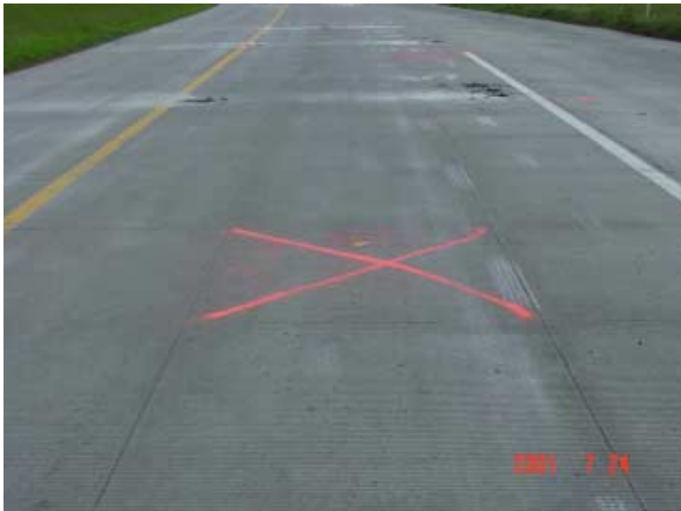
Figure 3.19 General View of Test Section S5E
