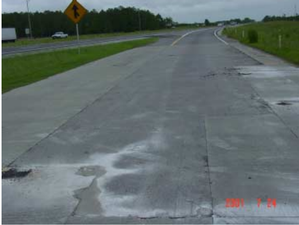
Figure 3.24 Asphalt Patch at the End of Section S6E
