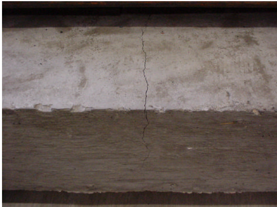
Figure B.11 – Specimen D Splitting failure
