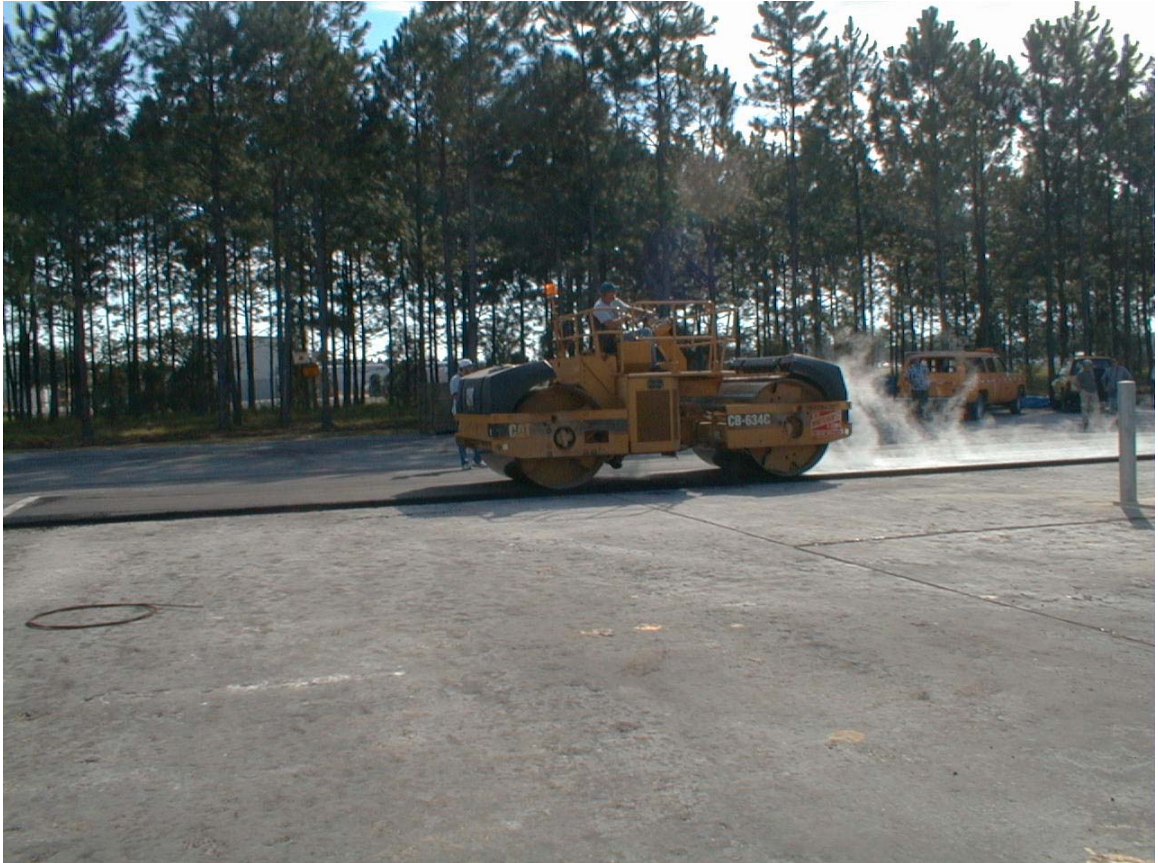
Figure 4.3 Photo of Steel-Wheel Roller used for compaction
