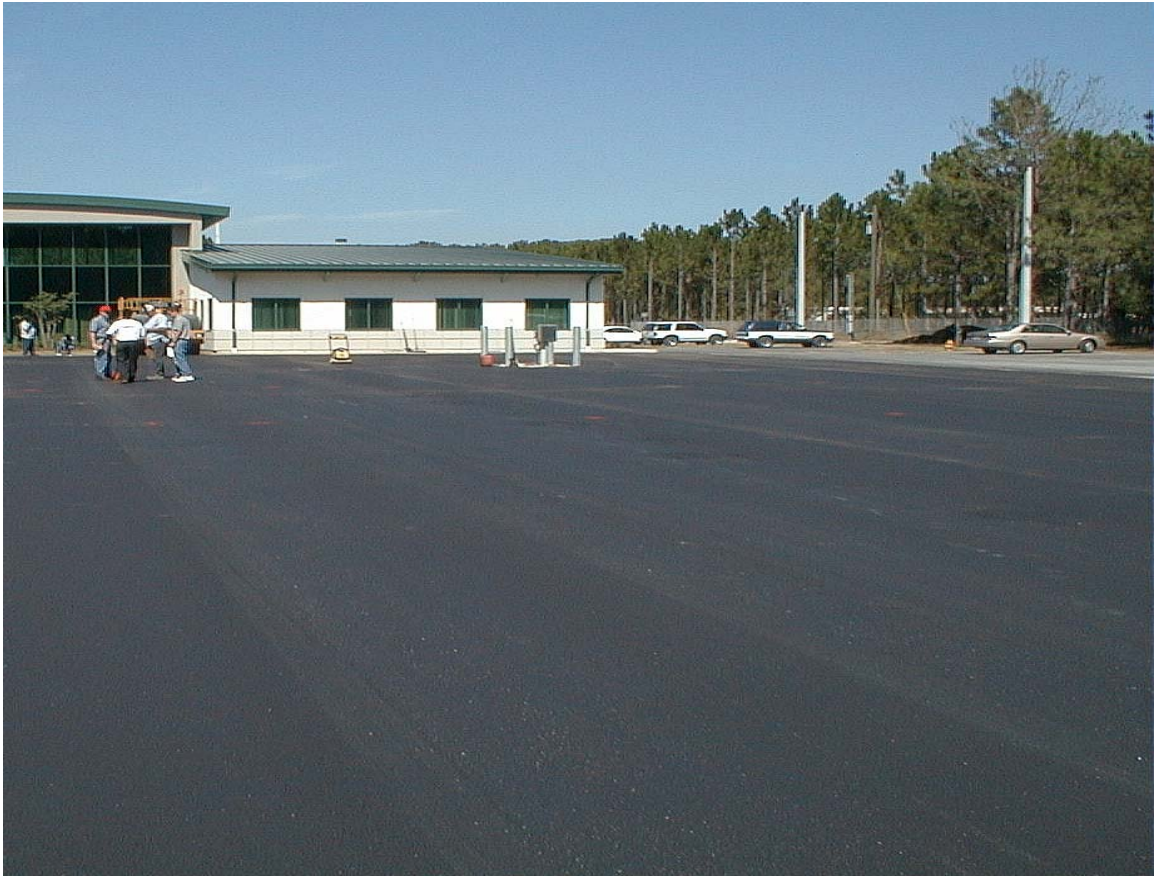
Figure 4.4 Photo of the Finished Test Track
