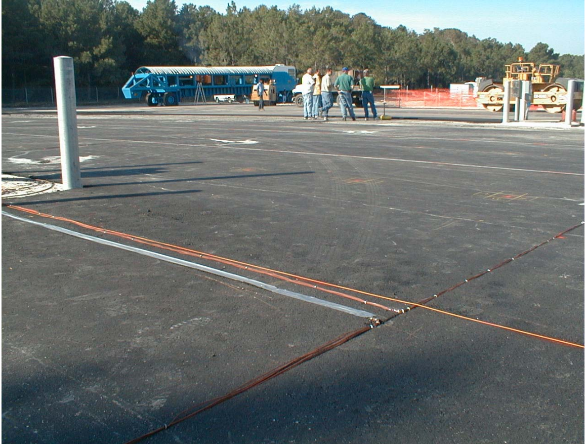
Figure 4.2 Photo of the thermocouples installed on the surface of the first lift of HMA
