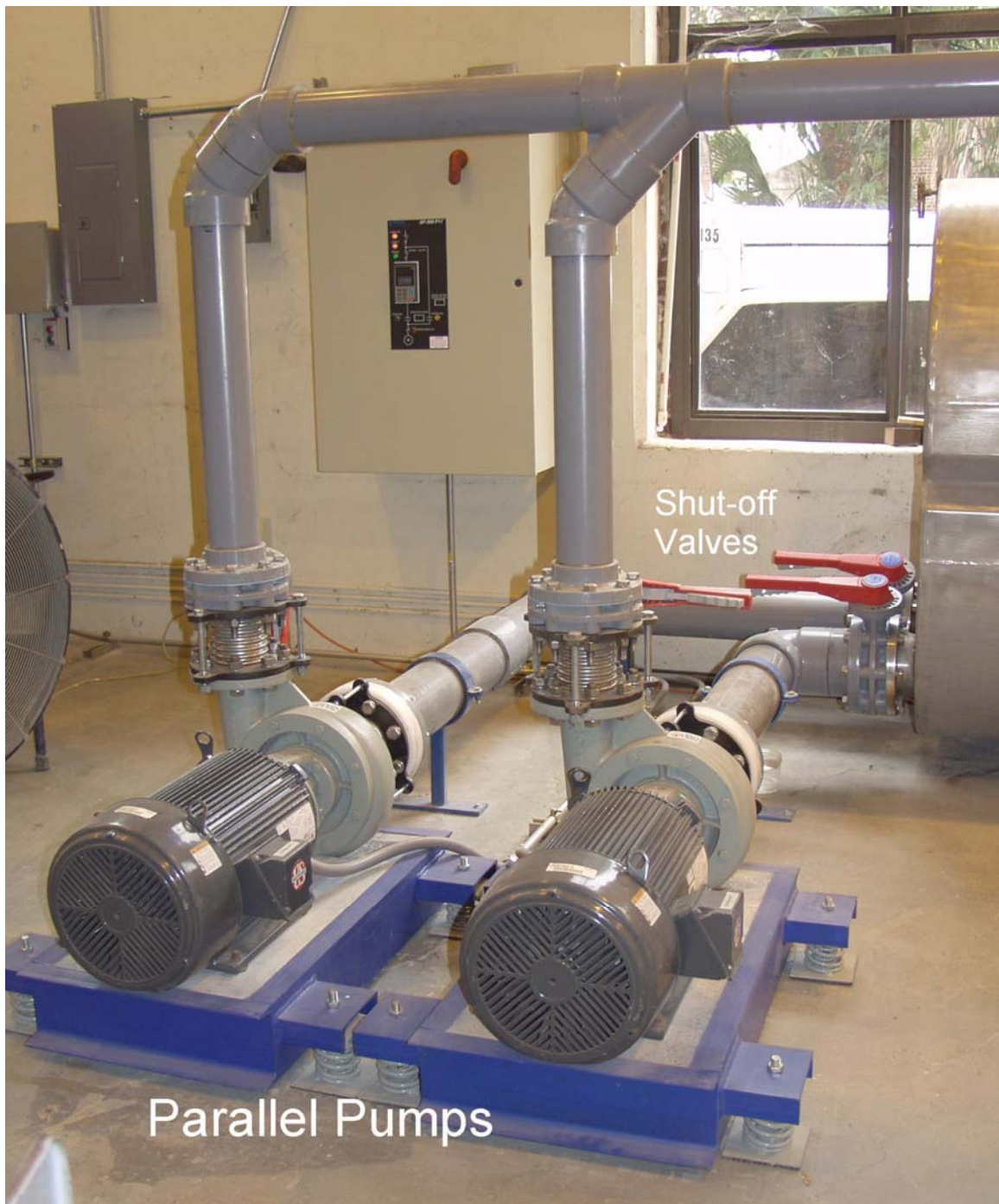
Figure IID - 2. The Pumps with Shut-Off Valves, Plumbing, and Pumps on the Inertial Bases.
