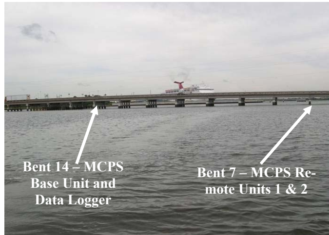
Figure 6: Dunn's Creek Bridge, Jacksonville Florida Field Evaluation Site.
