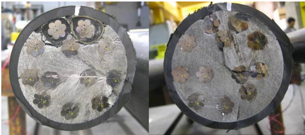
Figure 1.10 - Tendon 0B. L: Near S end. R: Near N end. Outlines of disbonding foam visible on two strands at S end.
