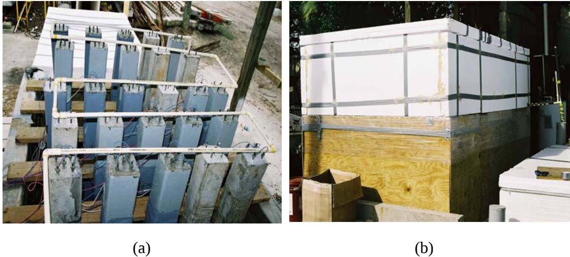
Figure 7.16 (a) Set Up of Piles; (b) Outside View of Hot Tank System
