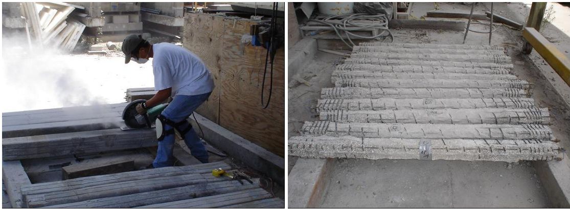
Figure 6.34 Breaking Surface Concrete to Retrieve Strands
