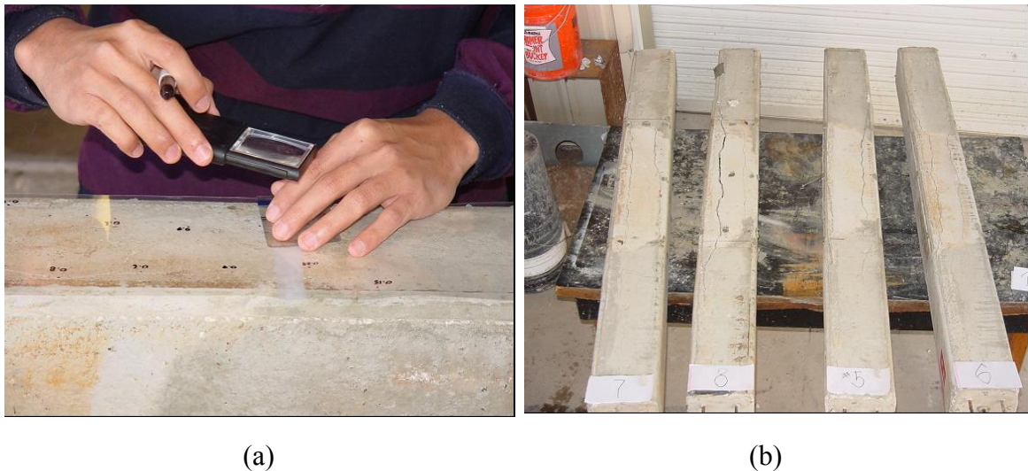
Figure 5.7 (a) Conducting Crack Survey; (b) Cracked Specimens
