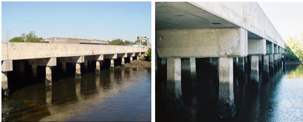
Figure 9.1 Allen Creek Bridge
