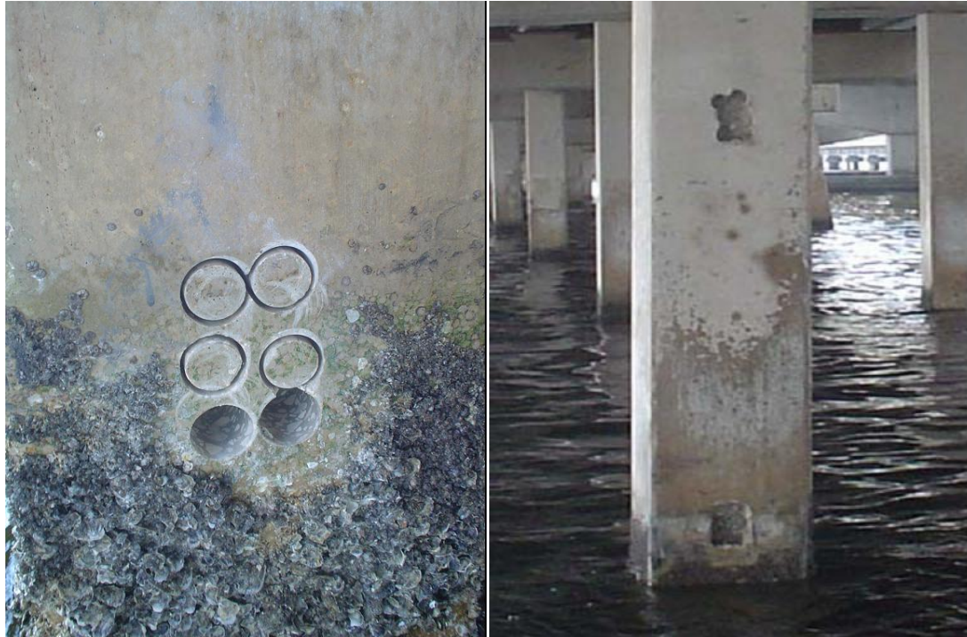
Figure 10.11 Coring for Commercial Probe Installation
