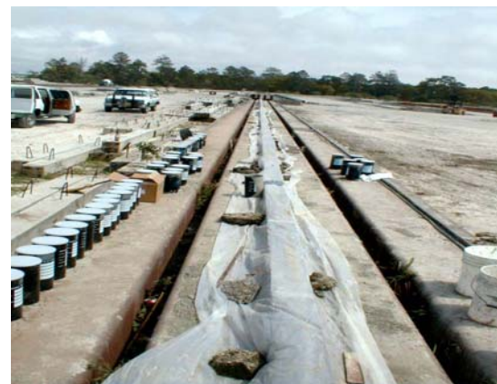
Figure 4.9 Surface Finishing and Curing.
