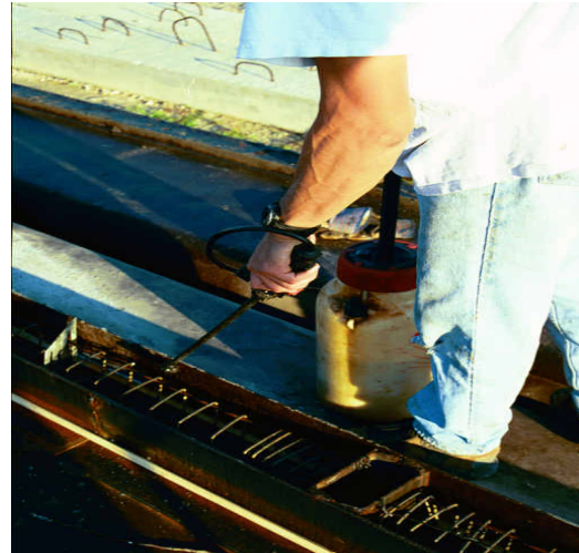
Application of Releasing Agent
