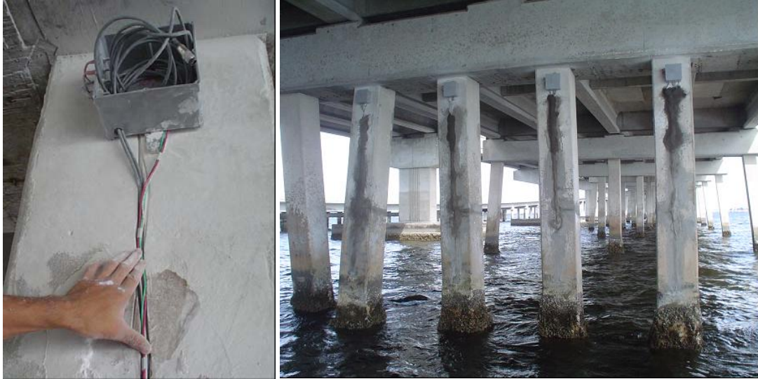
Figure 10.15 Installing Junction Box and Wiring
