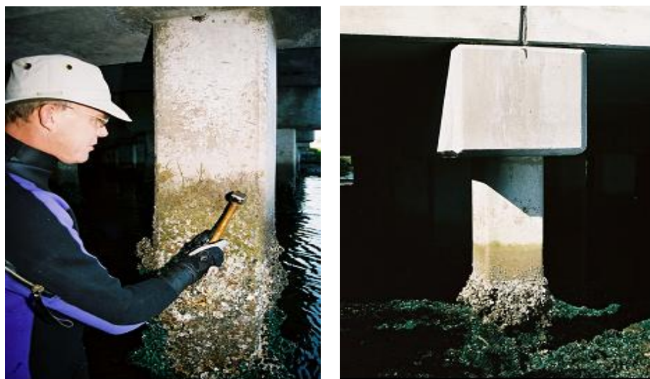
Figure 9.4 Checking for Delamination
