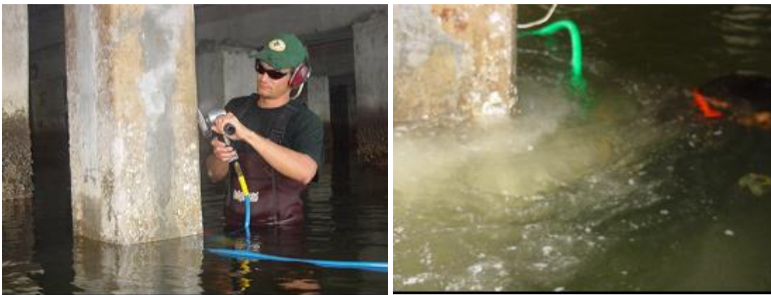
Figure 9.12 Grinding Edges
