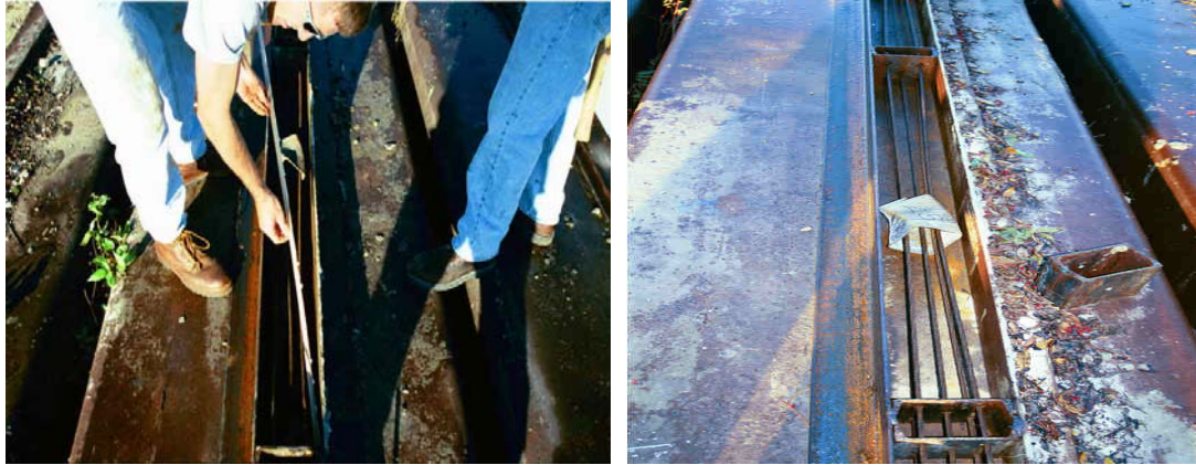
Figure 4.3 Wood Trims and Strands Positioning.
