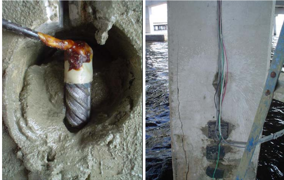
Figure 10.12 Rebar Probe Installation
