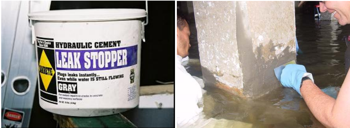
Figure 9.11 Filling Holes with Hydraulic Cement
