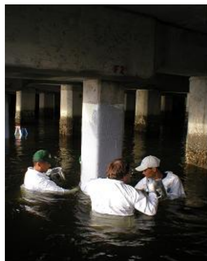
Figure 9.13 Underwater Wrapping (CFRP)
