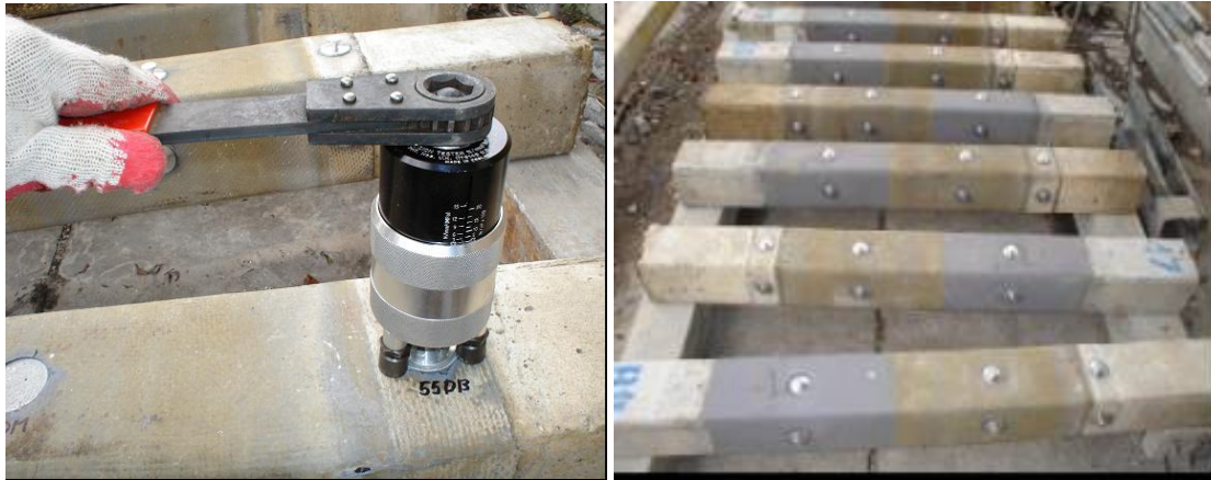
Figure 6.27 Performing Test with Elcometer (L) and Attached Dollies (R)
