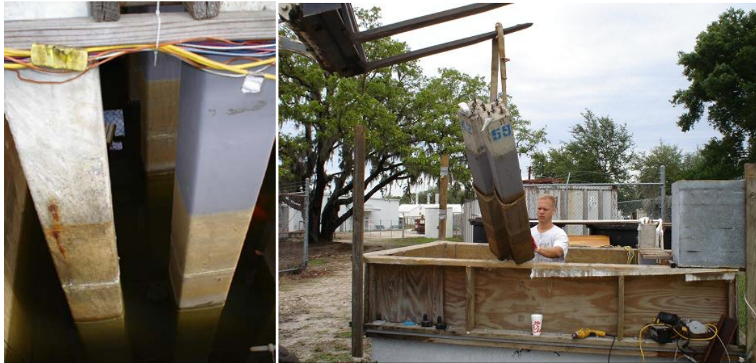
Figure 6.13 Cracks on the Unwrapped Specimen (L) and Removal of Specimens After Targeted Exposure
