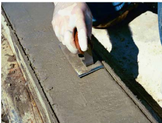
Figure 4.9 Surface Finishing and Curing.
