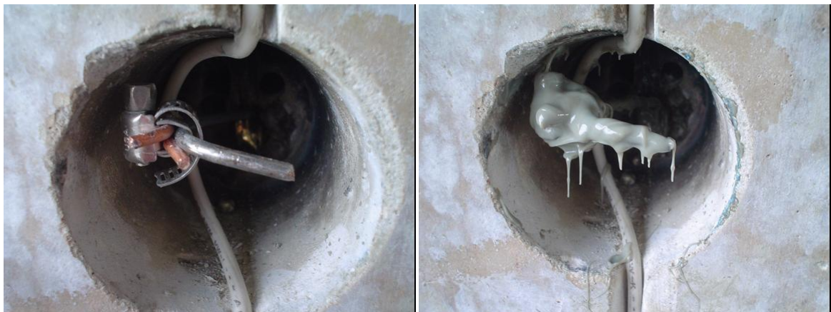
Figure 10.14 Connecting Grounding Cable to Steel
