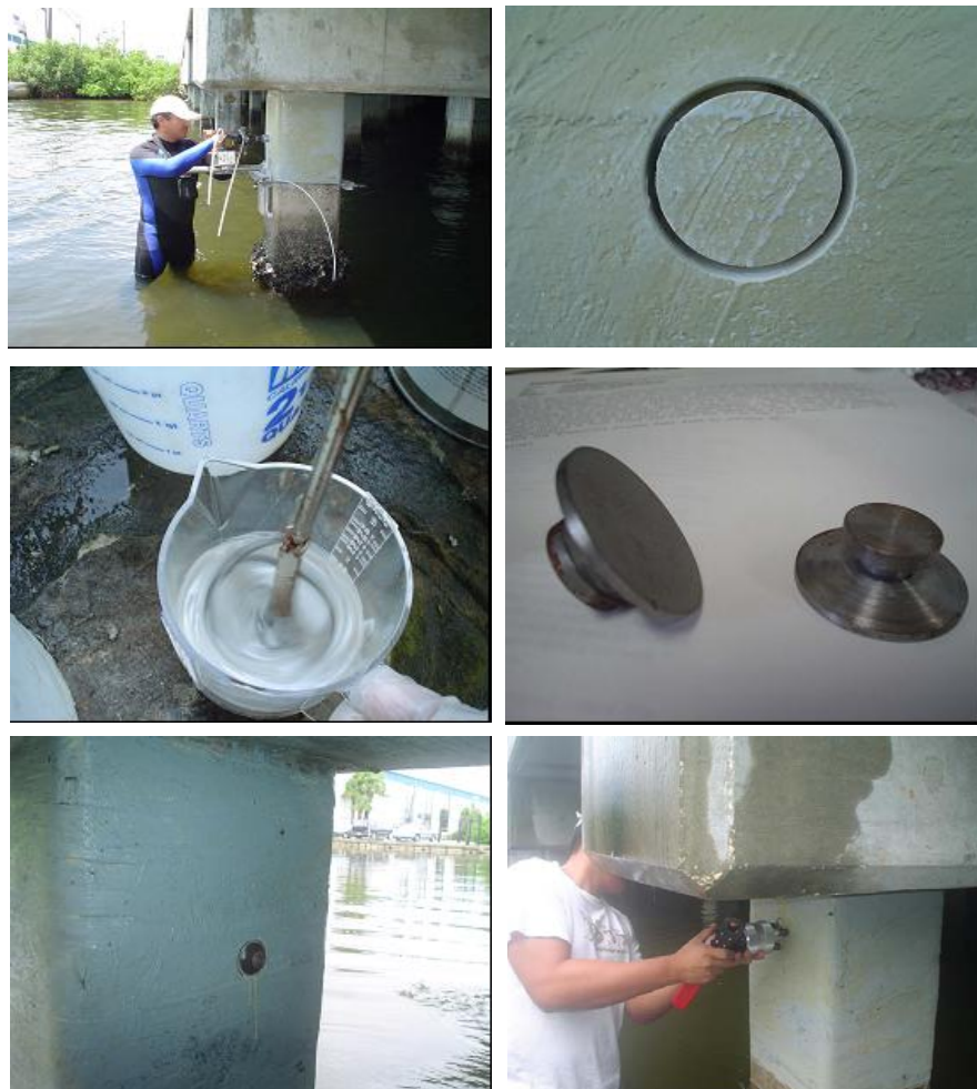
Figure 9.21 Pull-Out Test on Witness Panels.
