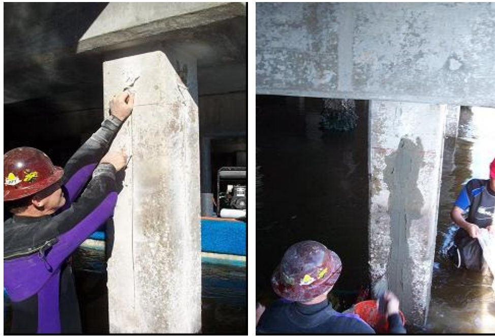
Figure 9.6 Installing Stainless Steel Rods
