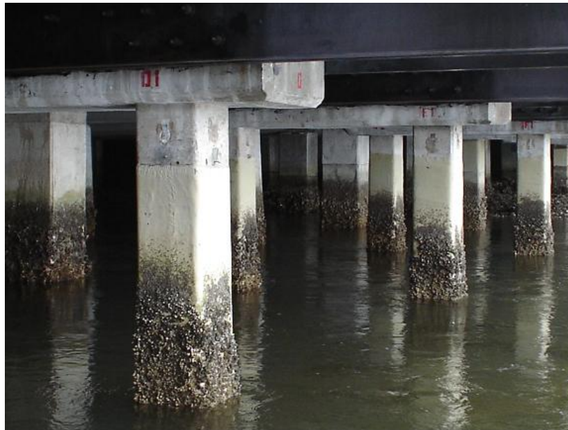
Figure 9.22 Wrapped Piles Covered with Marine Growth.
