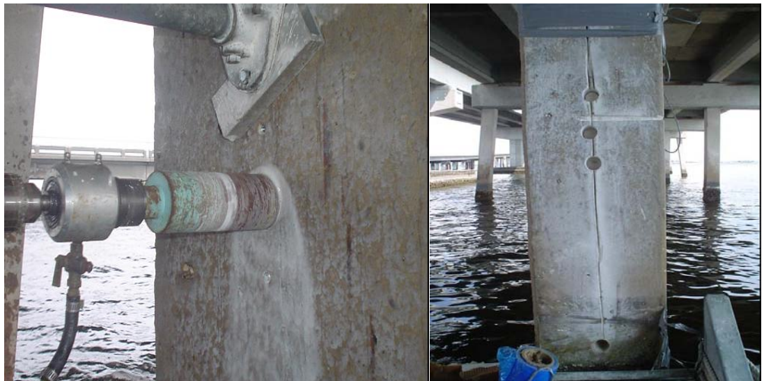
Figure 10.10 Coring Holes for Rebar Probe Installation
