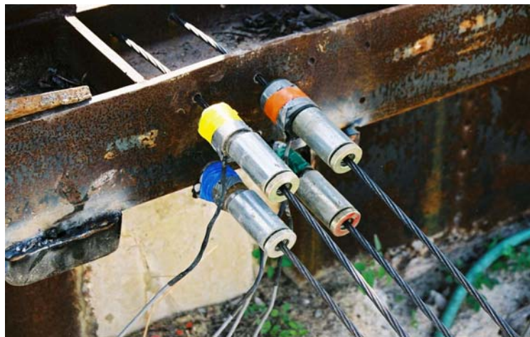
Figure 4.4 Load Cells and Prestressing Strands at Abutment.
