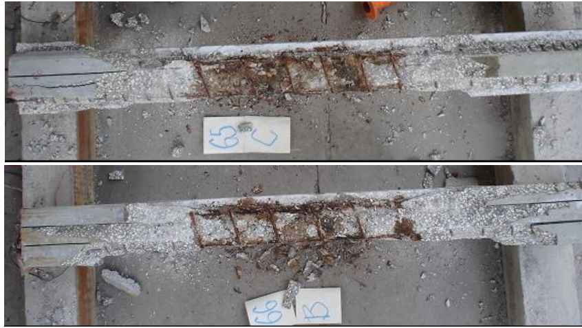
Figure 7.42 Distribution of Corrosion Product in #65 (T) and #66 (B)
