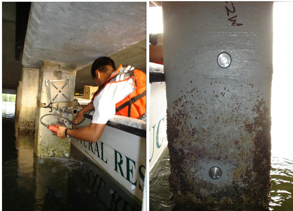
Figure 9.23 Bond Test in Progress.
