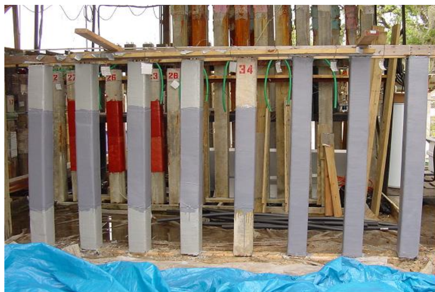
Figure 7.14 UV Paint Coated Piles
