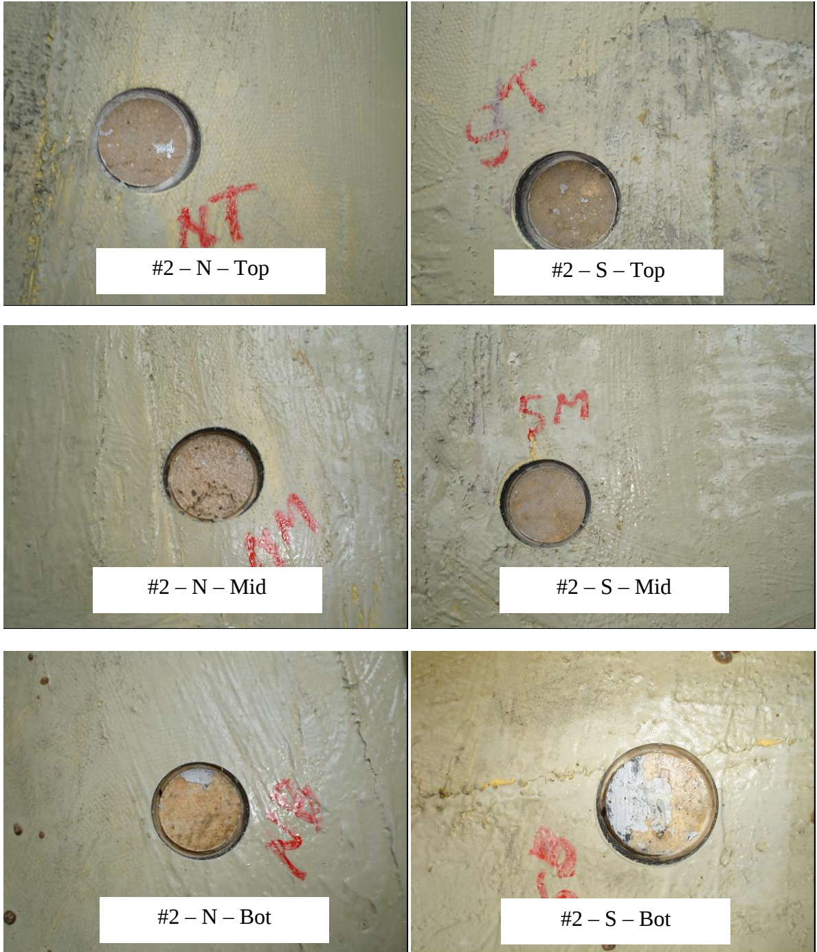
Figure 10.28 Bond Test on Pile2 (all epoxy failure)
