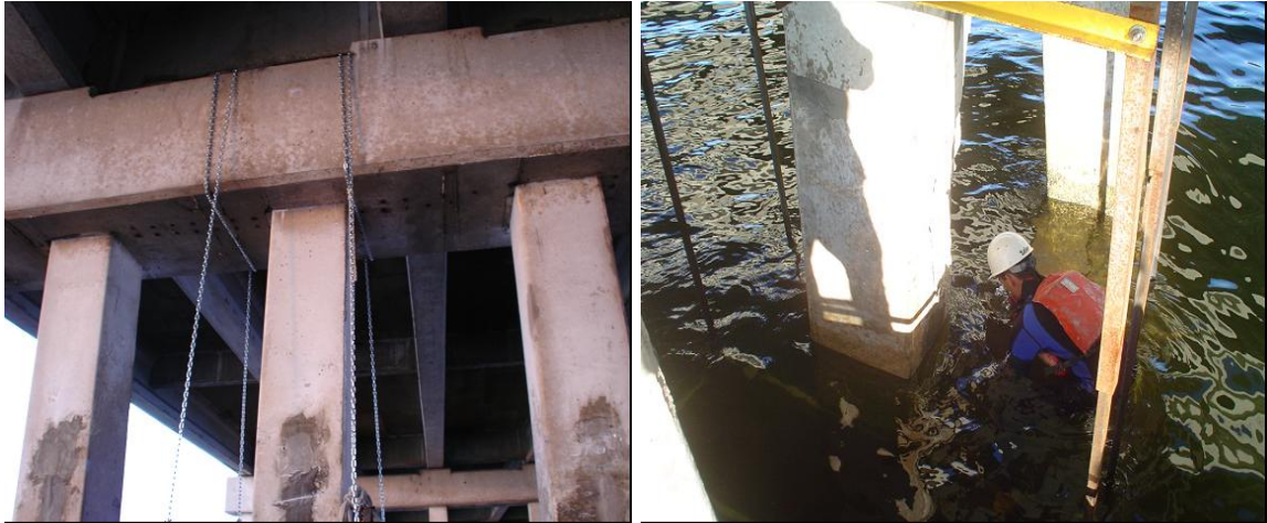
Figure 10.17 Installing Scaffolding Around a Pile
