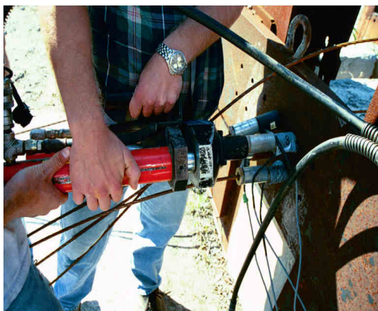
Figure 4.5 Prestressing Jack and Hydraulic Pump.
