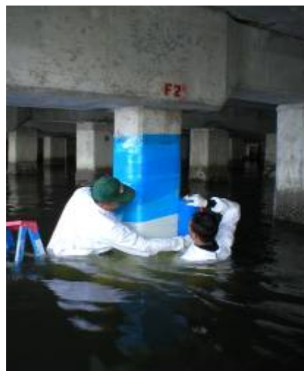
Figure 9.13 Underwater Wrapping (CFRP)
