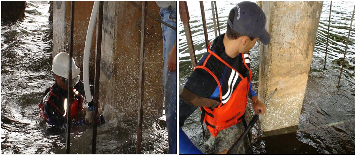
Figure 10.19 Surface Preparation of Piles
