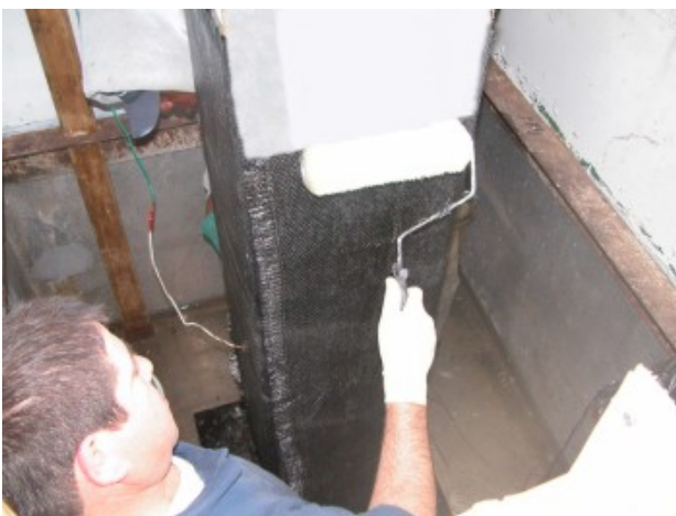
Figure 1.12 Carbon Wrap Application
