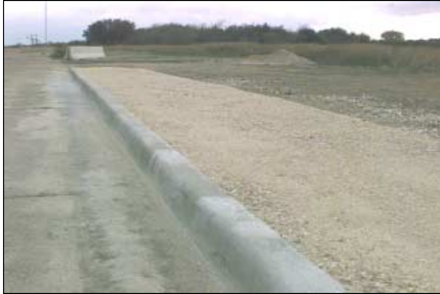
Fig. 1.14 – FDOT Type F curb (Texas Transportation Institute test site at College Station)
