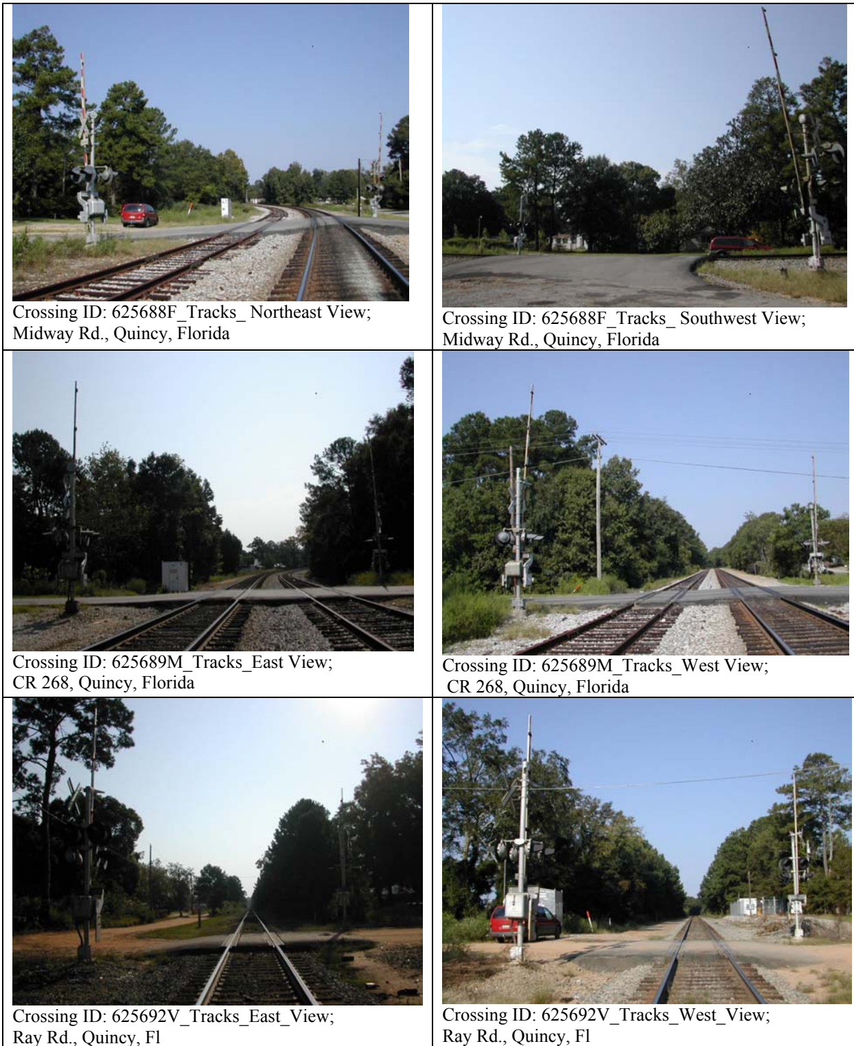
Figure 4.39. Inventory Photographs of Crossing IDs 625688F, 625689M, and 625692V
