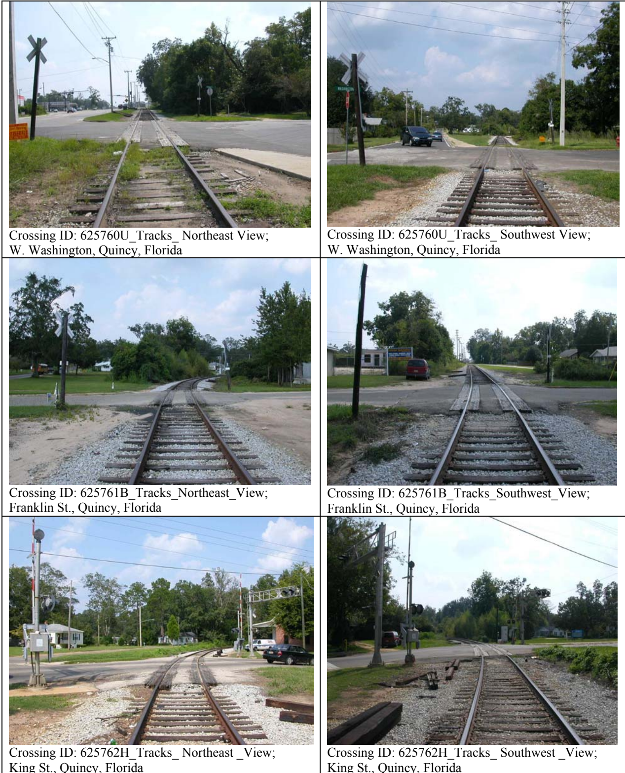
Figure 4.46. Inventory Photographs of Crossing IDs 625760U, 625761B, and 625762H
