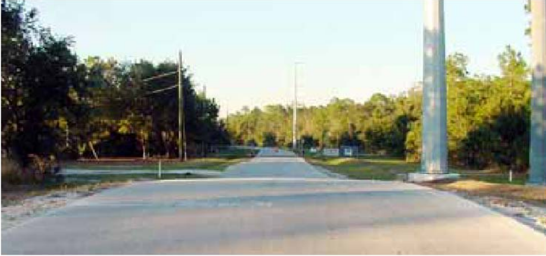
a. View Along Roadway
