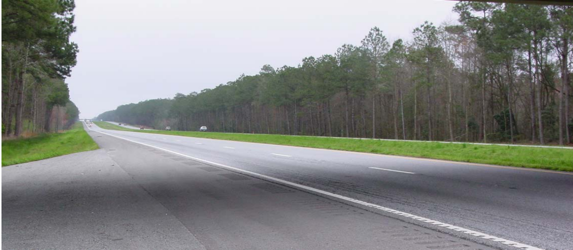
Figure B-4: Site 9928 Eastbound lanes on the left
