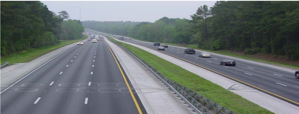
Figure B-2: Site 9904 Northbound lanes on the right
