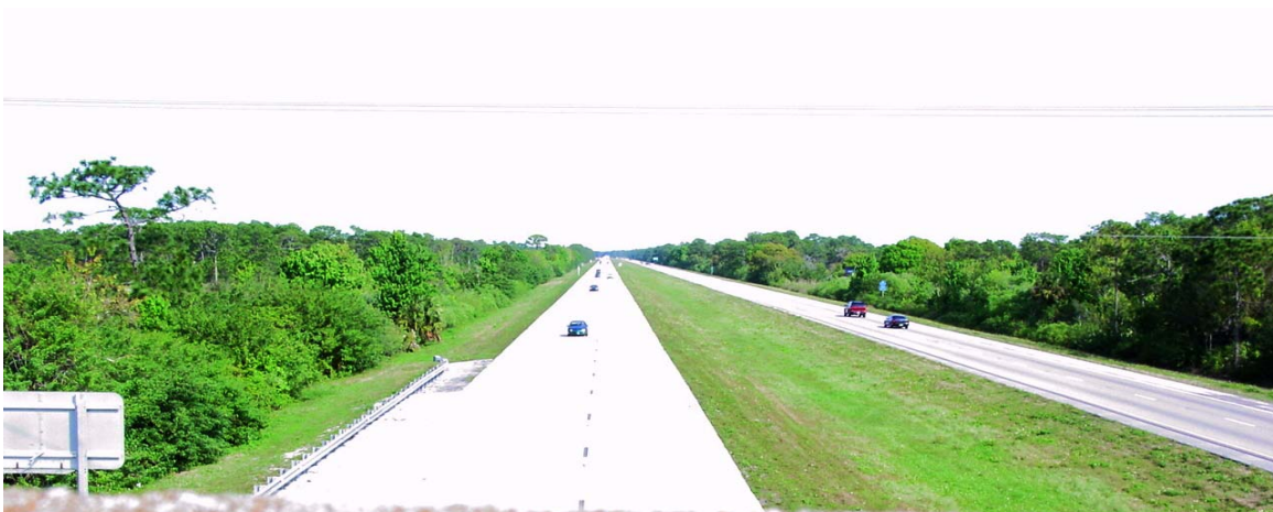
Figure B-6: Site 9919 Northbound lanes on the right
