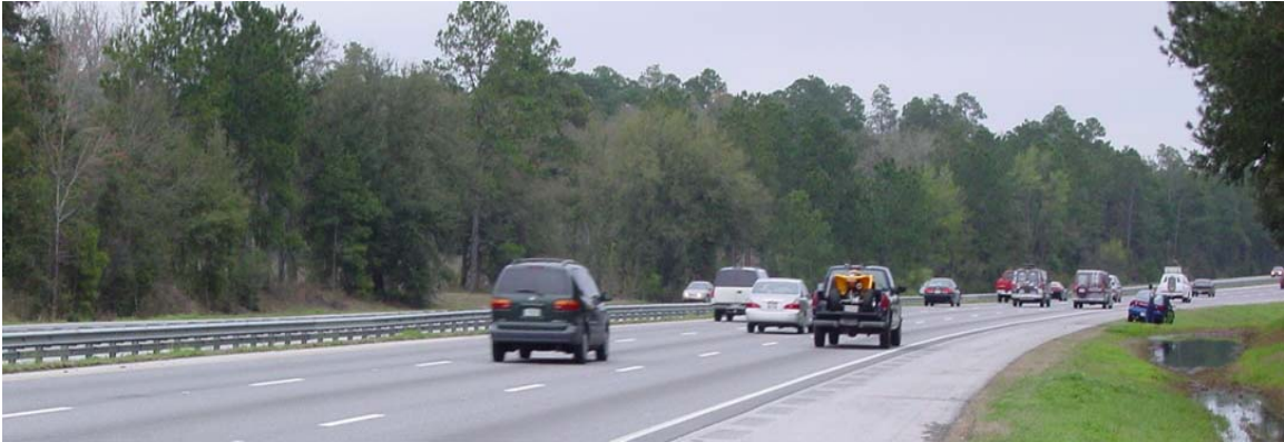
Figure B-1: Site 320 Northbound lanes on the right
