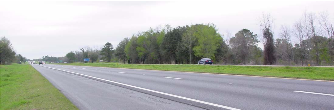
Figure B-3: 9901 Eastbound lanes on the left
