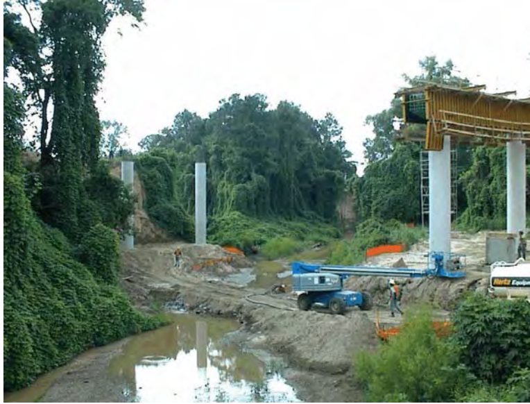
Figure 4-137 Natchez: Production bridge bents.
