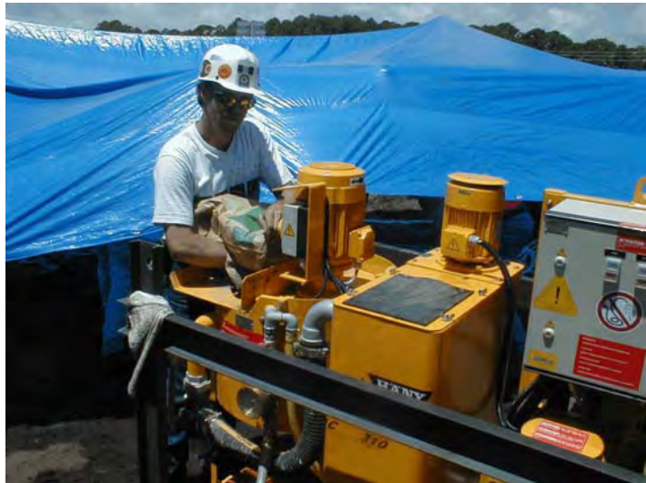
Figure 4-14 PGA Blvd: Post grouting using neat cement with w/c ratio of 0.50.
