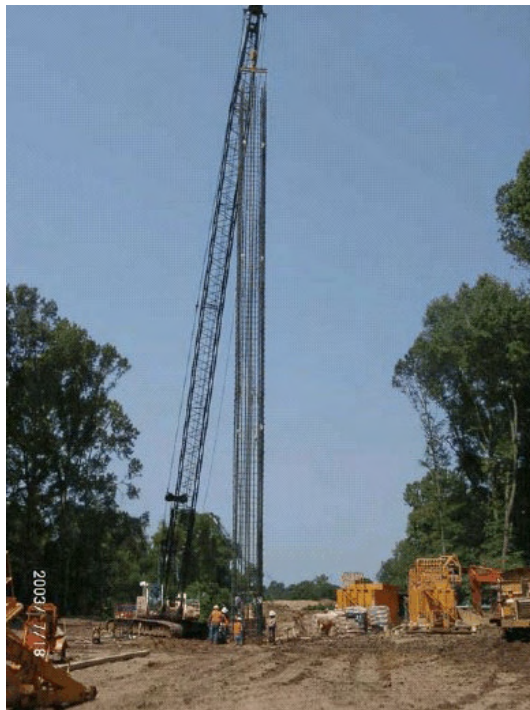
Figure 4-136 Natchez: Bent 8 cage placement.
