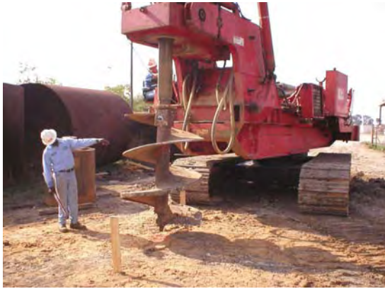
Figure 4-89 TexDOT Demo: Drilling of 48" diameter test shafts.
