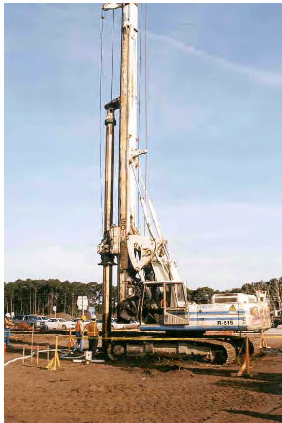
Figure 4-6 PGA Blvd: Drilling of test shafts.
