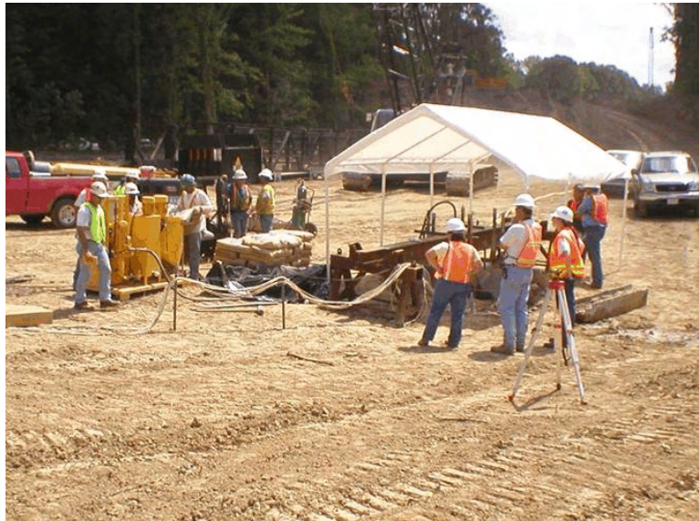
Figure 4-121 Natchez: Post grout setup and testing.
