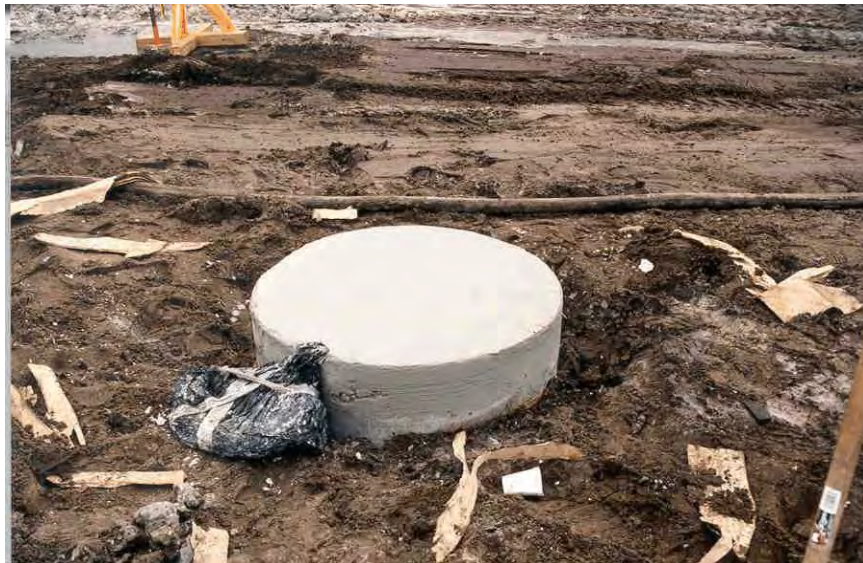
Figure 4-10 PGA Blvd: Control test shaft.
