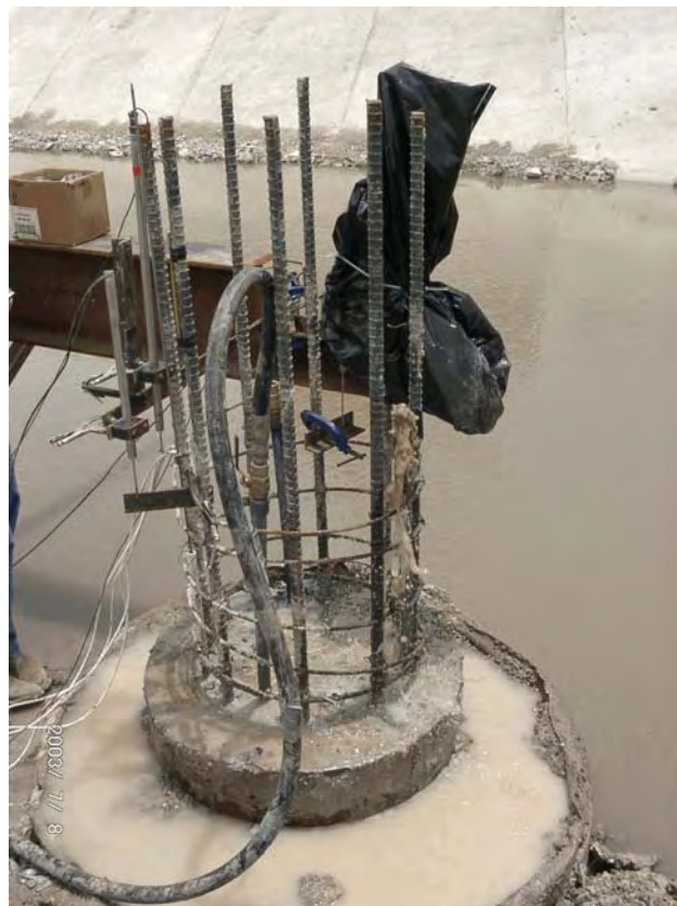
Figure 4-153 FM 507: Grouting of the west shaft.
