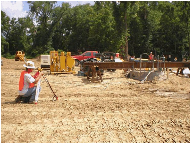
Figure 4-120 Natchez: Field survey during post grouting (quality assurance testing of post grouting).
