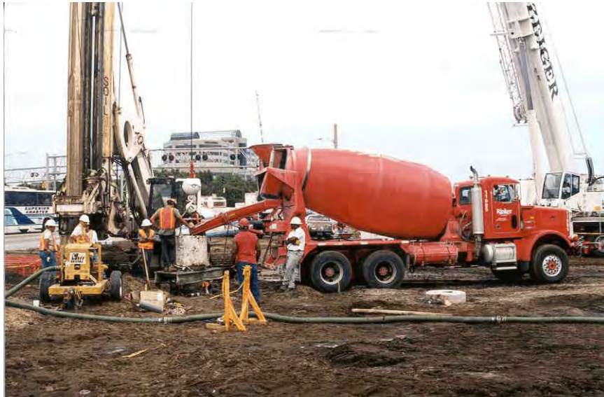
Figure 4-9 PGA Blvd: Concrete pour of test shafts.
