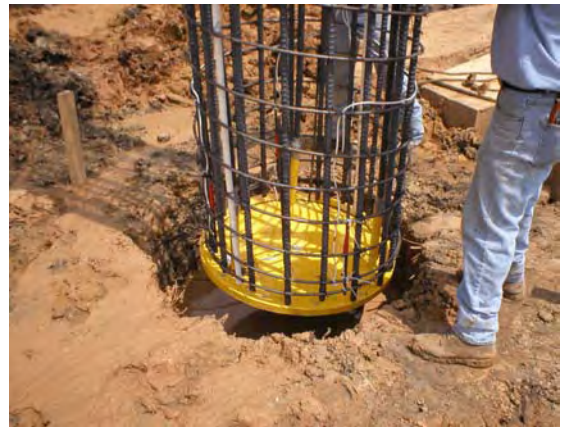
Figure 4-90 TexDOT Demo: Reinforcement cage placement.
