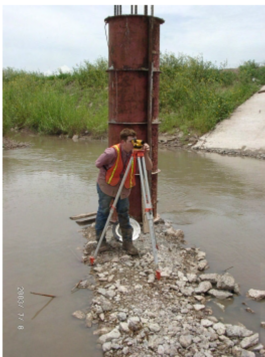
Figure 4-155 FM 507: Field surveying during grouting.
