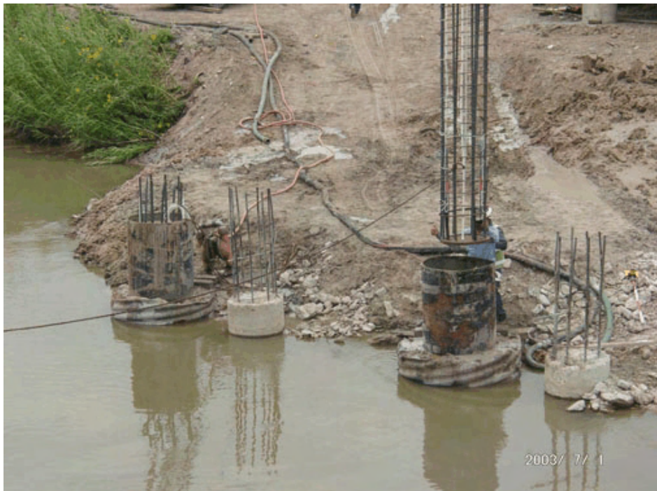
Figure 4-149 FM 507: East shaft cage placement.
