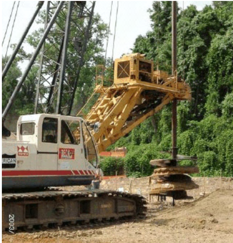
Figure 4-111 Natchez: Crane mounted drill rig.
