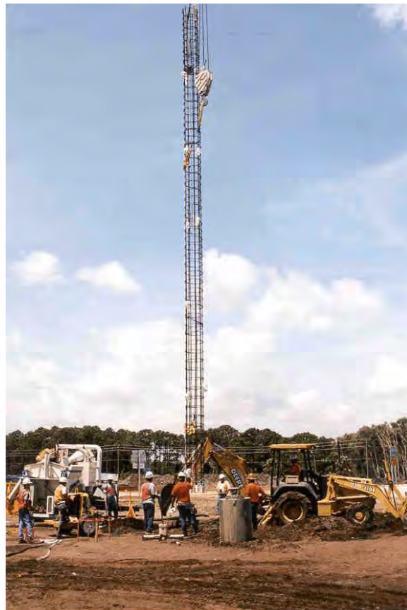
Figure 4-8 PGA Blvd: Reinforcement cage placement.
