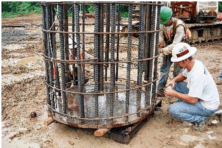
Figure 4-116 Natchez: Grout plate installation.
