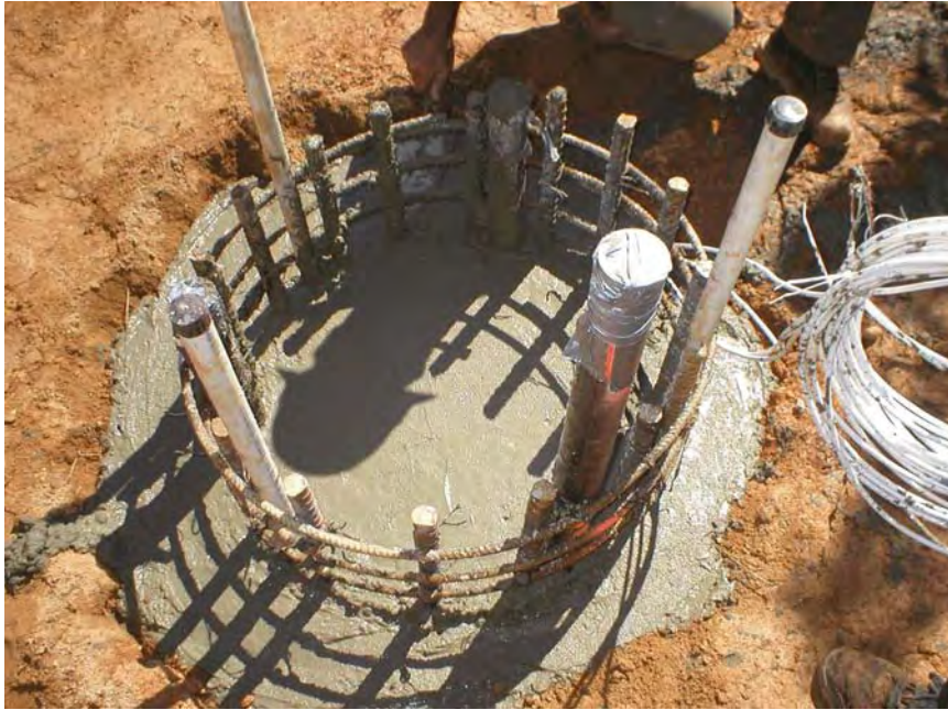
Figure 4-53 NGES Auburn: Top of shaft finishing.
