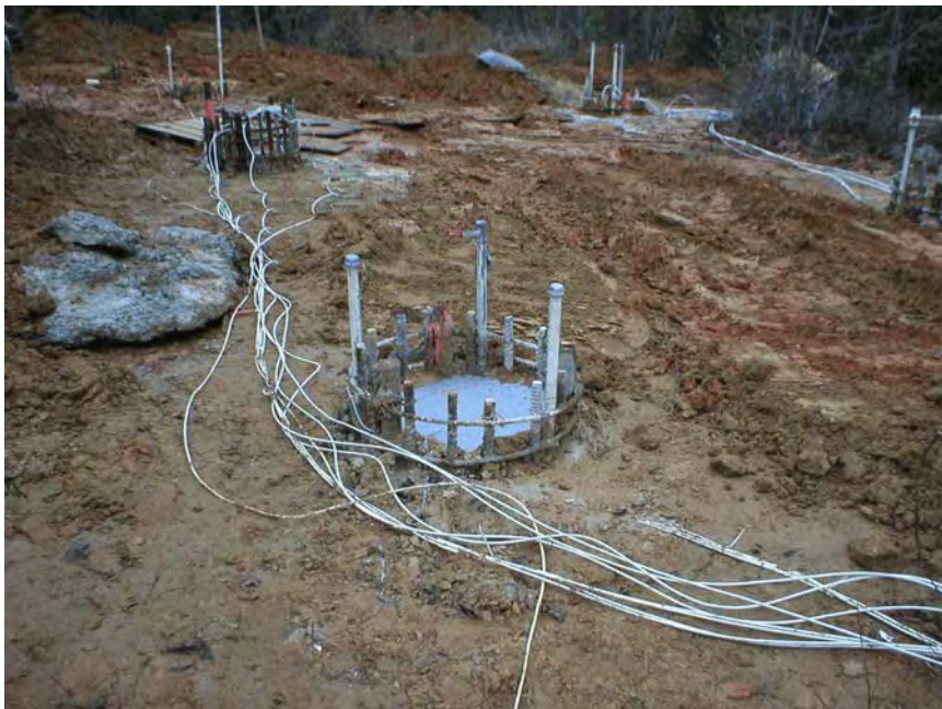
Figure 4-54 NGES Auburn: Test shafts.
