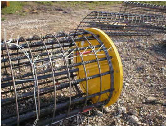
Figure 4-88 TexDOT Demo: Grout plates and strain gages installed.
