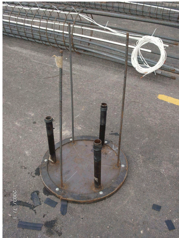
Figure 4-147 FM 507: 24" grout plate.
