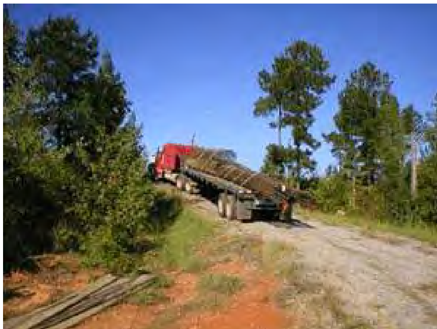
Figure 4-46 NGES Auburn: Reinforcement cages.
