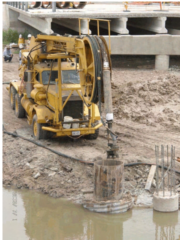
Figure 4-143 FM 507: Submersible de-sanding pump.
