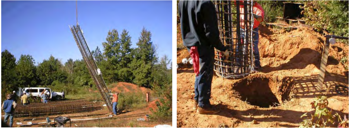
Figure 4-51 NGES Auburn: Reinforcement cage installation.
