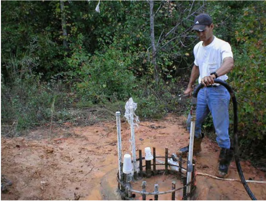
Figure 4-57 NGES Auburn: Flushing grout lines.
