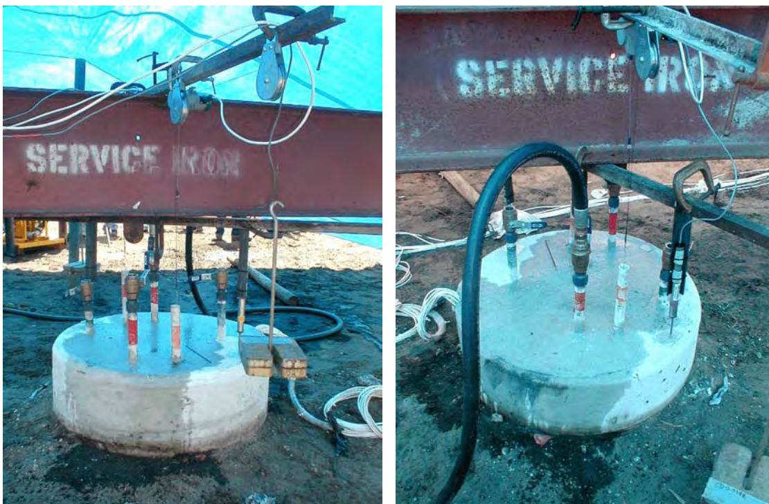
Figure 4-11 PGA Blvd: Post grout instrumentation setup.
