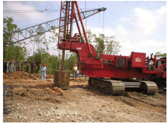
Figure 4-89 TexDOT Demo: Drilling of 48" diameter test shafts.
