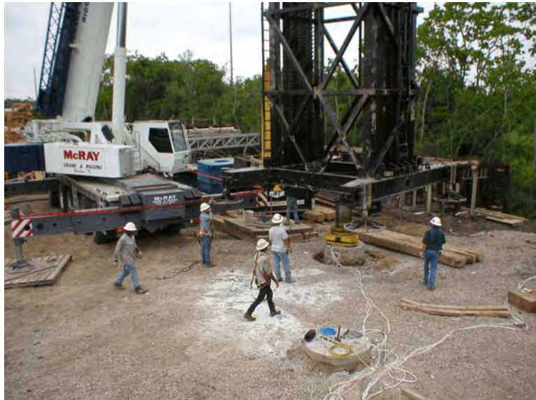
Figure 4-103 TexDOT Demo: Statnamic setup
