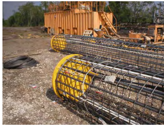
Figure 4-88 TexDOT Demo: Grout plates and strain gages installed.
