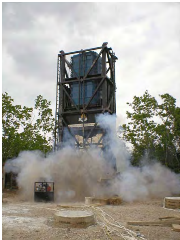
Figure 4-104 TexDOT Demo: Statnamic load test
