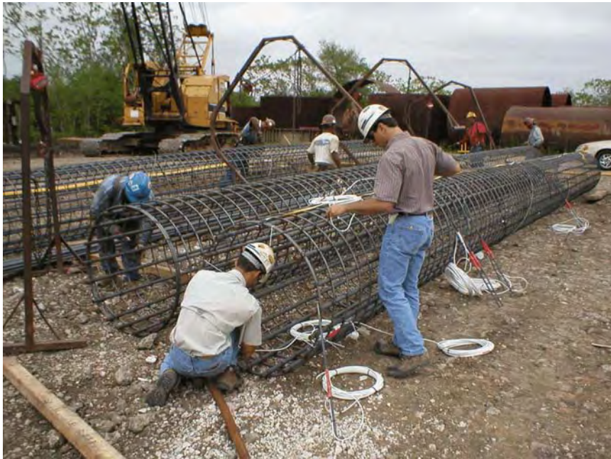
Figure 4-85 TexDOT Demo: Strain gage installation.
