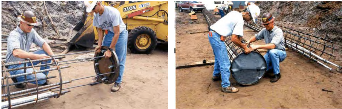
Figure 4-5 PGA Blvd: Installation of grout plate.
