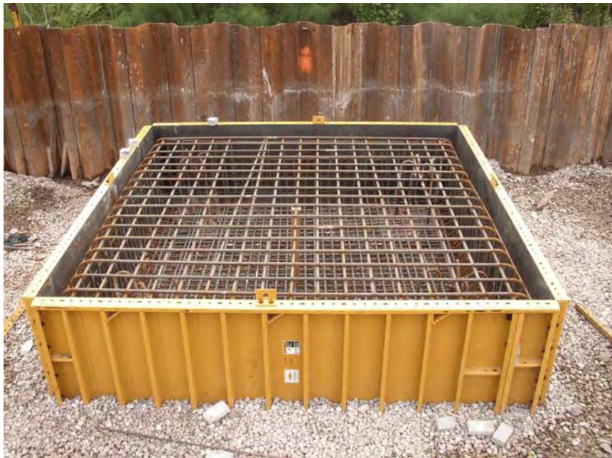
Figure 4-28 PGA Blvd: Pier 2 pile cap reinforcement.
