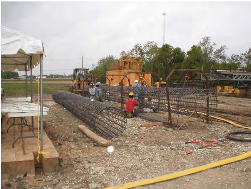
Figure 4-84 TexDOT Demo: Reinforcement cage construction.
