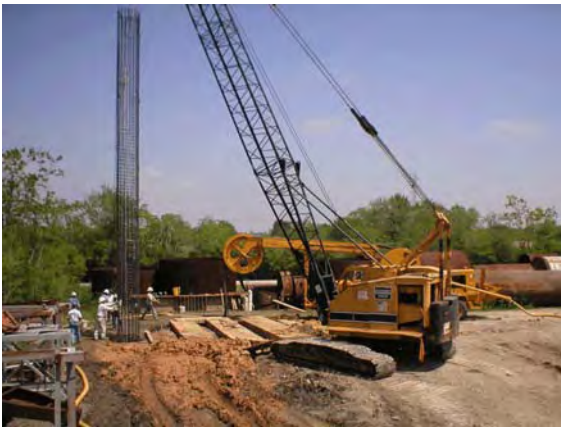
Figure 4-90 TexDOT Demo: Reinforcement cage placement.
