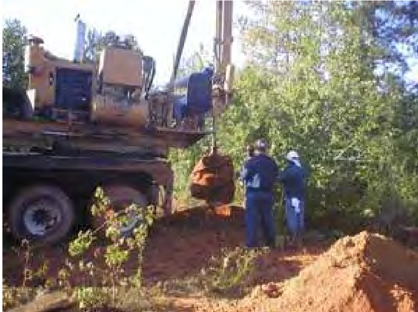
Figure 4-49 NGES Auburn: Drilling of 42" diameter test shafts.
