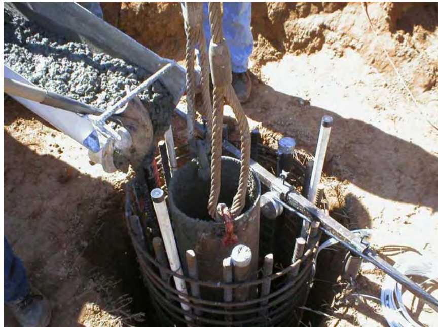
Figure 4-52 NGES Auburn: Drilled shaft concrete pour.
