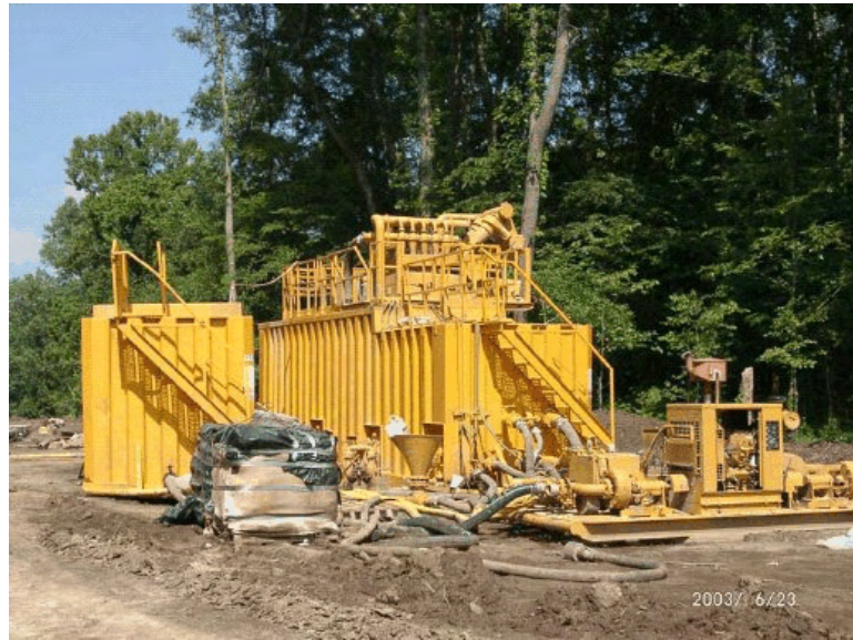
Figure 4-113 Natchez: Slurry tank and de-sanding unit.
