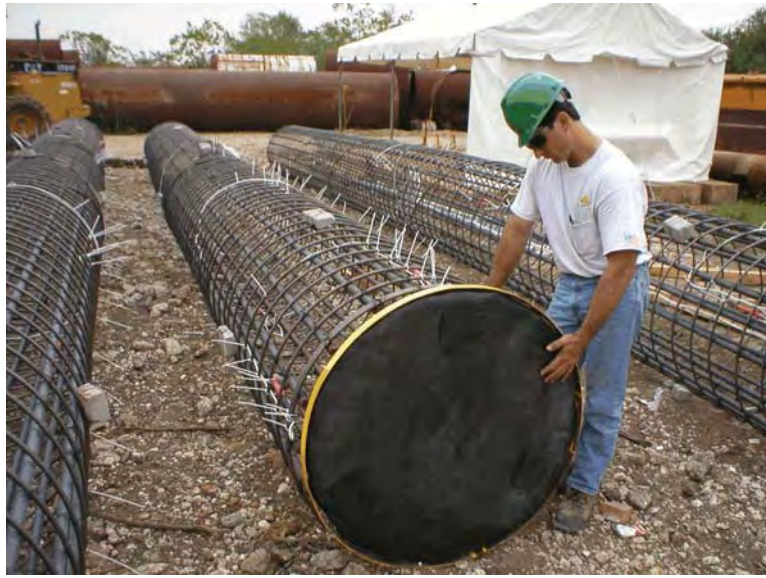
Figure 4-87 TexDOT Demo: Grout plate installation.
