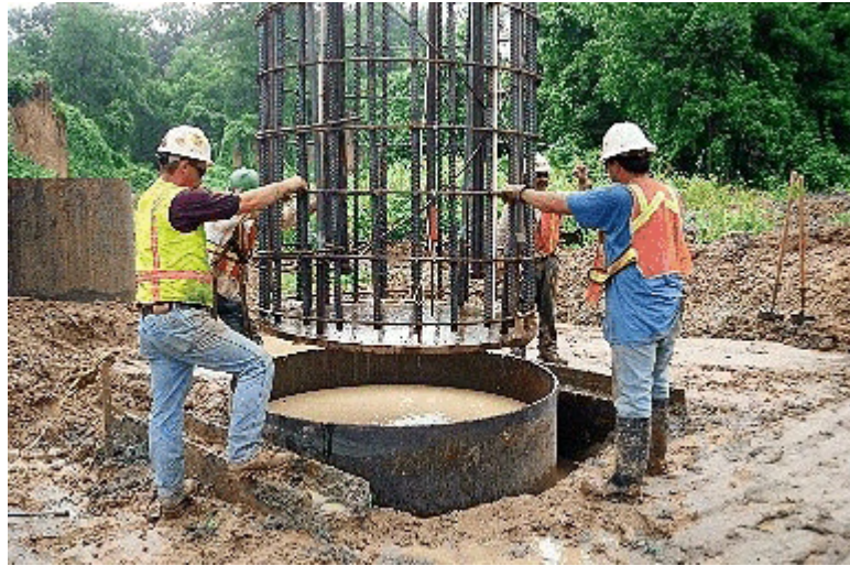
Figure 4-117 Natchez: Reinforcement cage installation.
