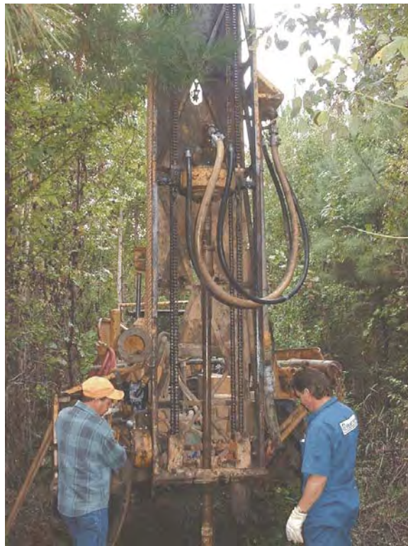
Figure 4-110 Natchez: SPT testing.
