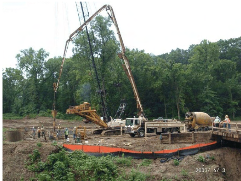
Figure 4-118 Natchez: Concrete placement with a pump truck.
