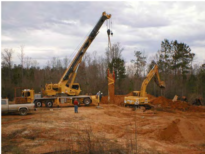
Figure 4-78 NGES Auburn: Shaft extraction.
