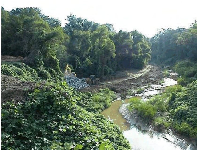
Figure 4-134 Natchez: Production site preparation.
