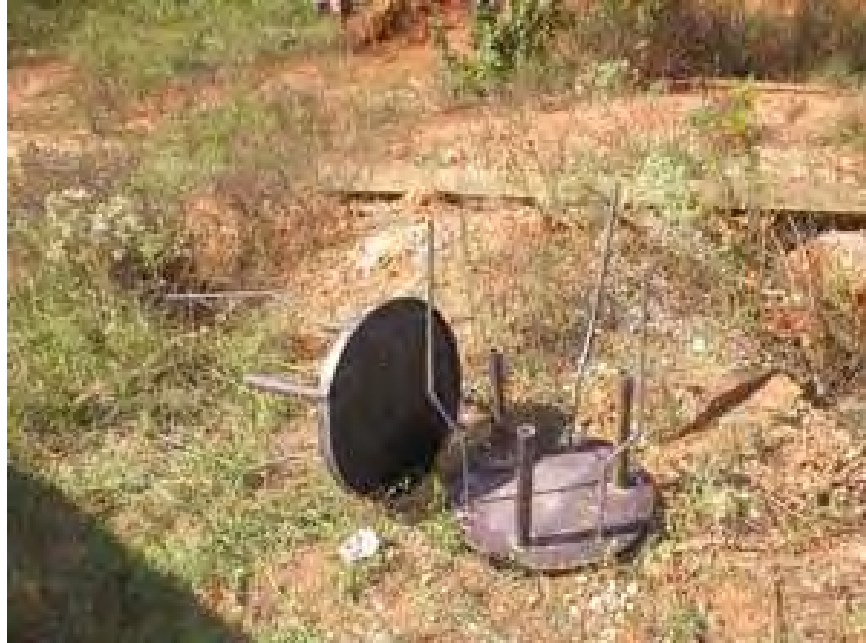
Figure 4-47 NGES Auburn: 24" diameter grout plates.
