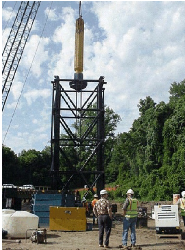
Figure 4-129 Natchez: Statnamic load test setup.
