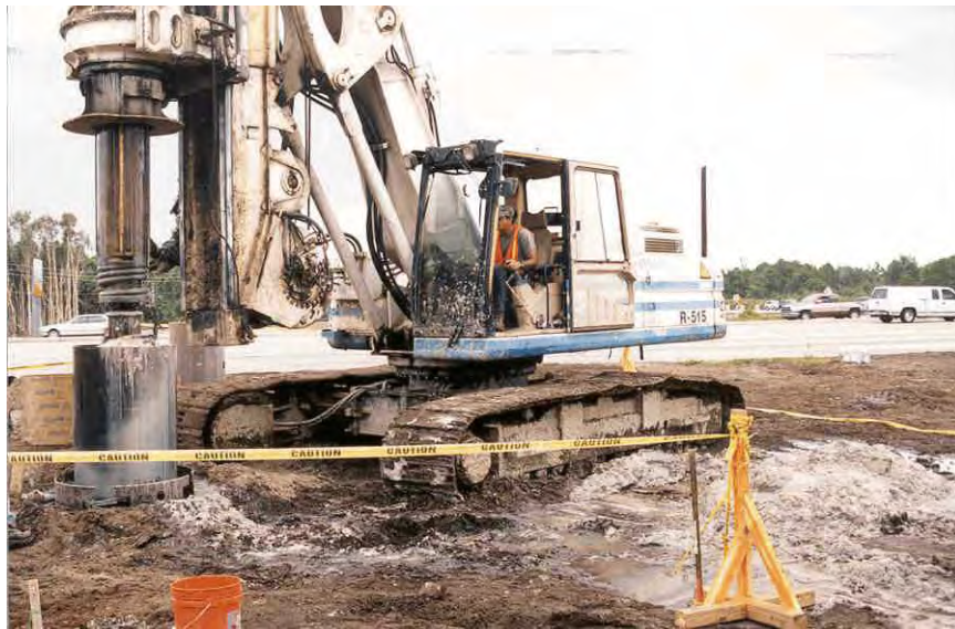
Figure 4-7 PGA Blvd: Clean-out of bottom to ensure cleanliness of bottom prior to cage placement.
