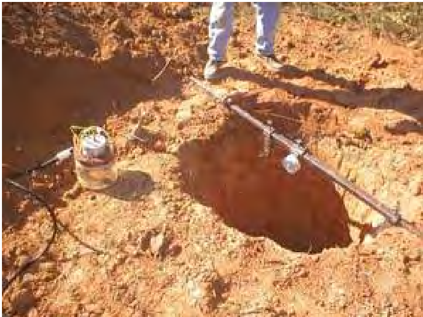
Figure 4-50 NGES Auburn: FDOT Borescope inspection.
