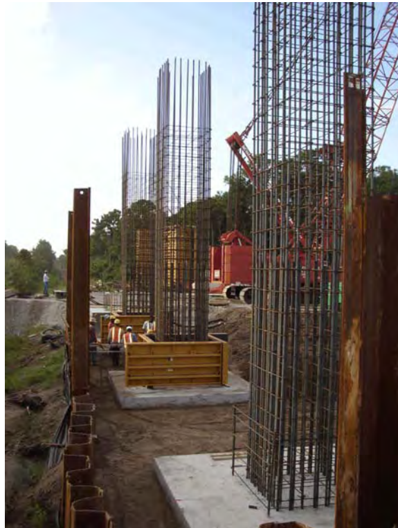
Figure 4-30 PGA Blvd: Pier 2.
