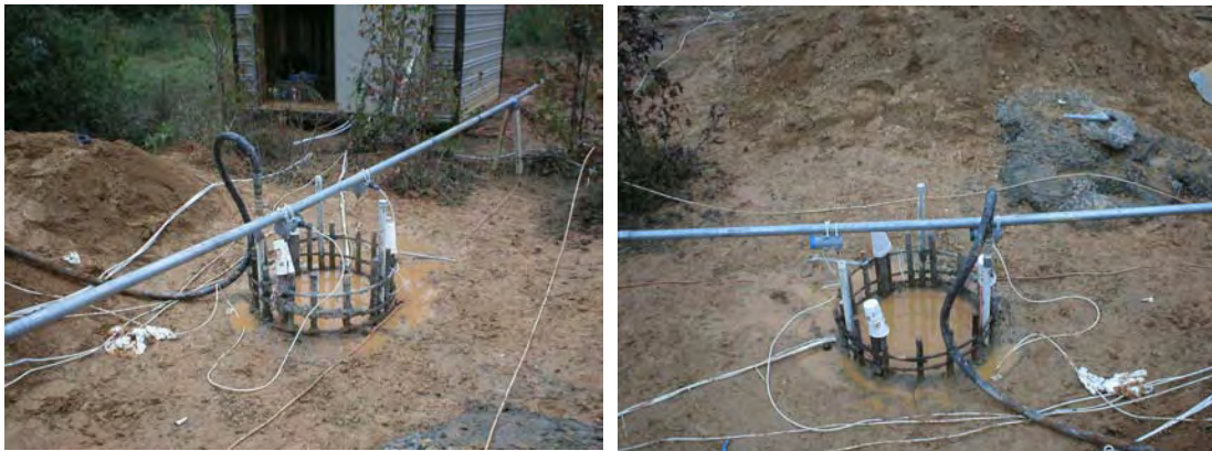
Figure 4-58 NGES Auburn: Post grouting test setup.
