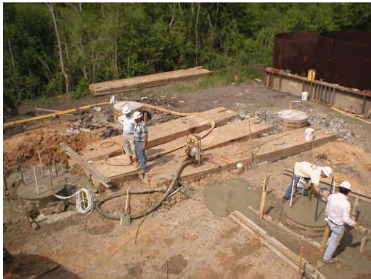
Figure 4-92 TexDOT Demo: Test site.
