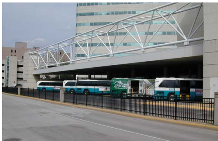
Angled bus bays at the GTC.
