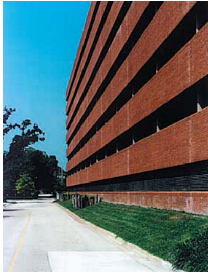
Parking Garage: Auto-Oriented Façade
