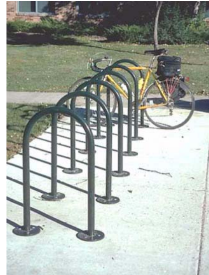
The standard inverted U type bike rack supports the bike frame at two locations and allows users to secure their bikes with either a cable or U type lock. Source: (13).
