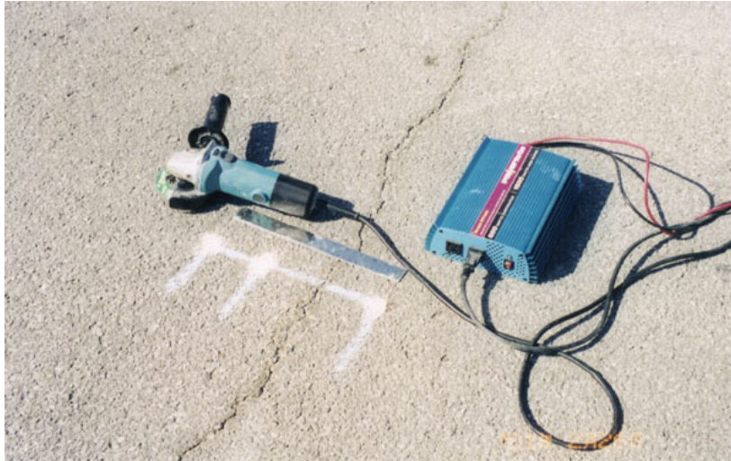
Figure 5-4. Pavement Surface Polish for Impact Echo Testing
