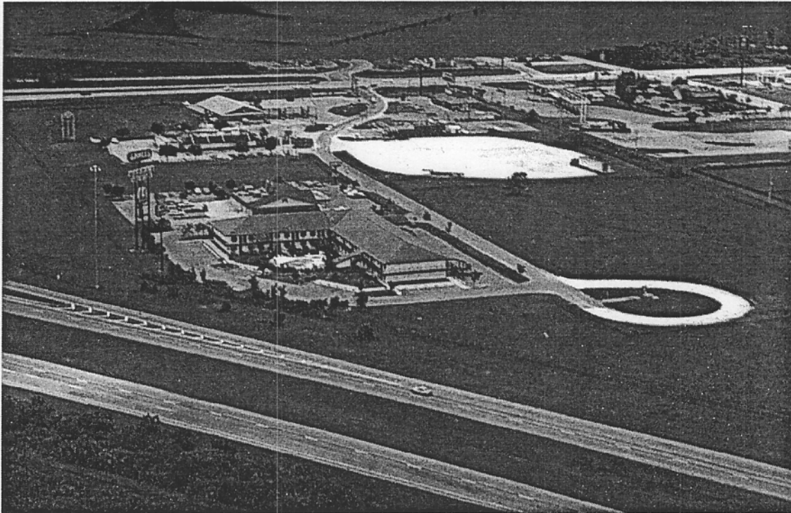
Figure 13 Internal Access Road Near Interchange
