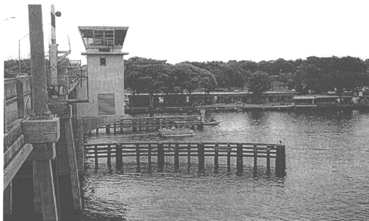
Figure 1.1. Fender Systems Currently Used by FDOT
