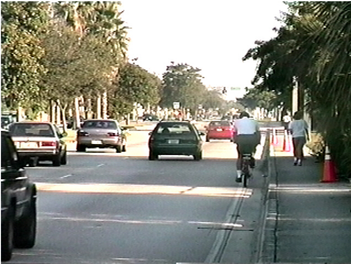
Figure 1. Before condition with 14-foot wide curb lane.
