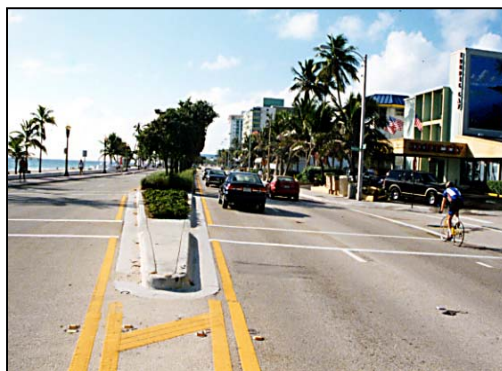
Figure 3. SR A1A, the ‘Strip’ after the conversion to 11- and 3- foot lanes
