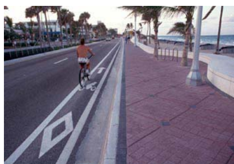
Figure 4. SR A1A with three-foot marked bike lanes.
