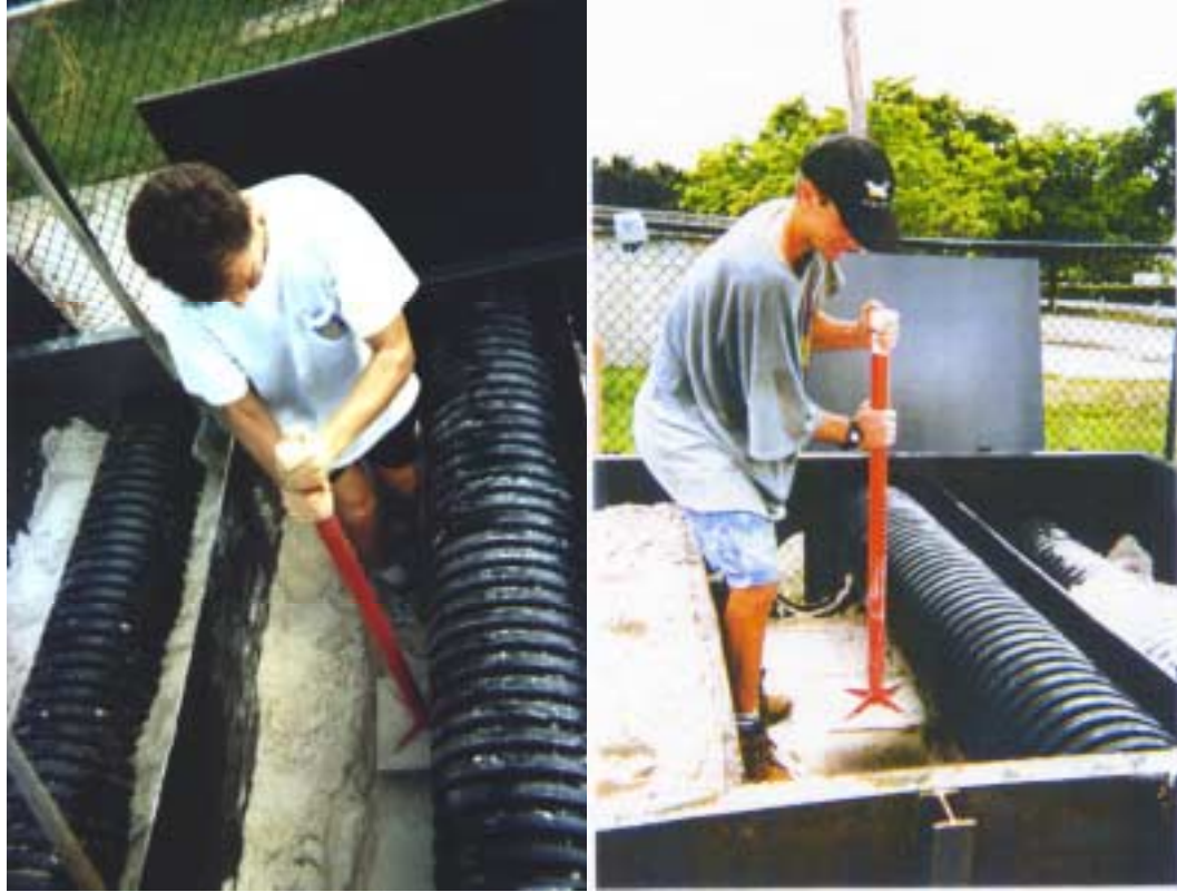
Fig. 4.2 and 4.3 Compaction below the pipe
