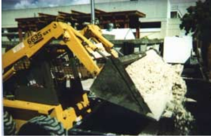
Fig. 3.20 Filling up of the soil chamber
