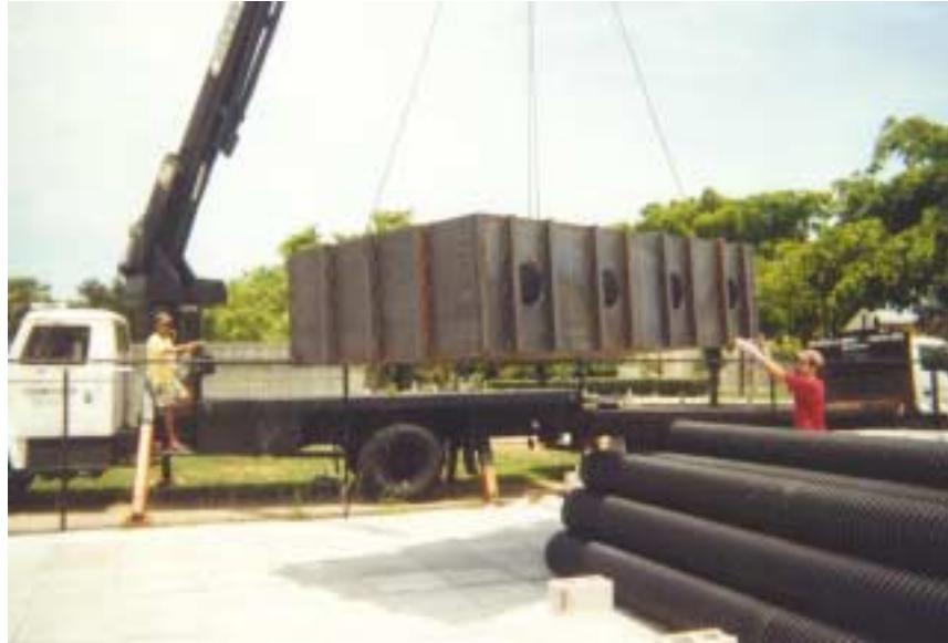
Fig. 3.18 Delivery of soil chambers
