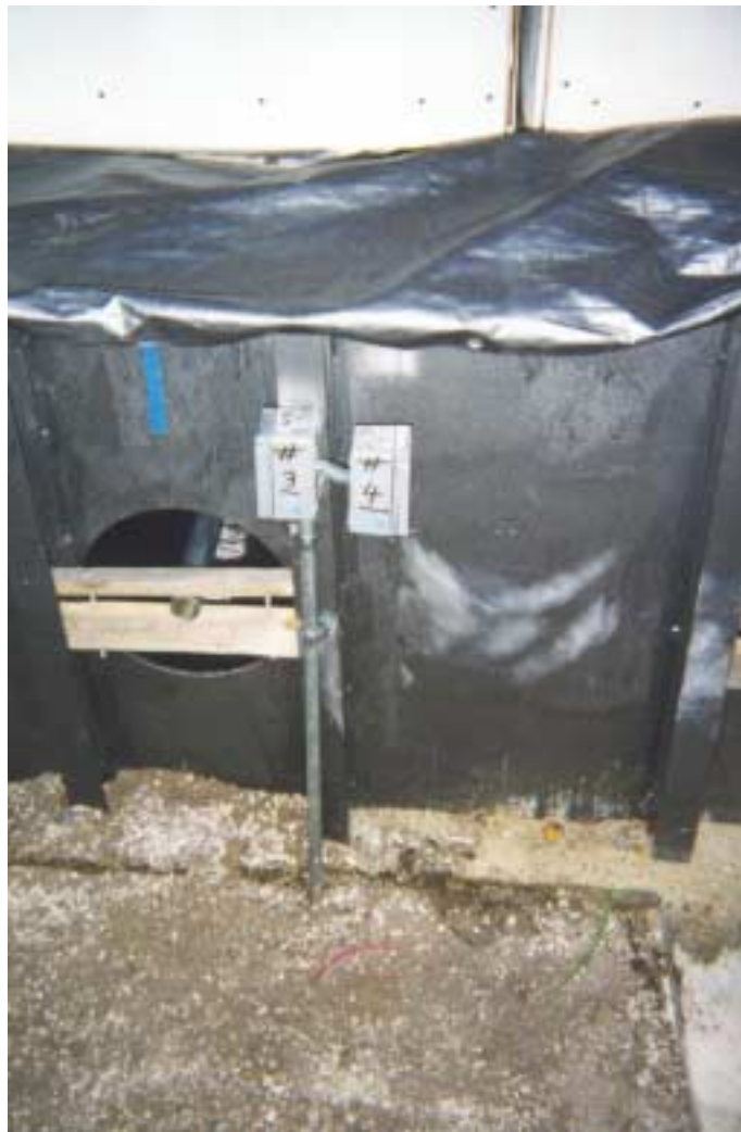
Fig. 3.16 Installation of the power line (2x 4 outlets) for the heaters
