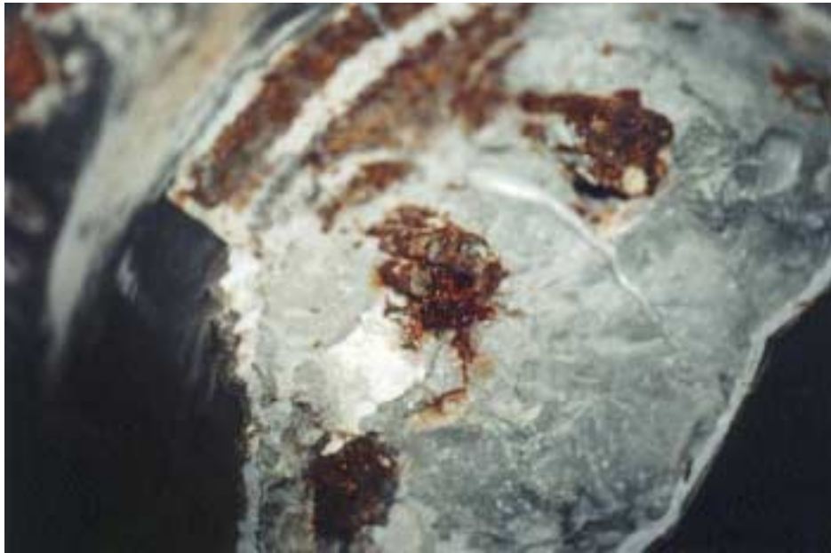
Figure 8. Photograph of the exposed end of a tendon anchorage.
