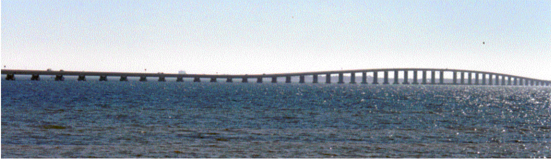
Figure 1. View of the Mid Bay Bridge, Destin, Florida.
