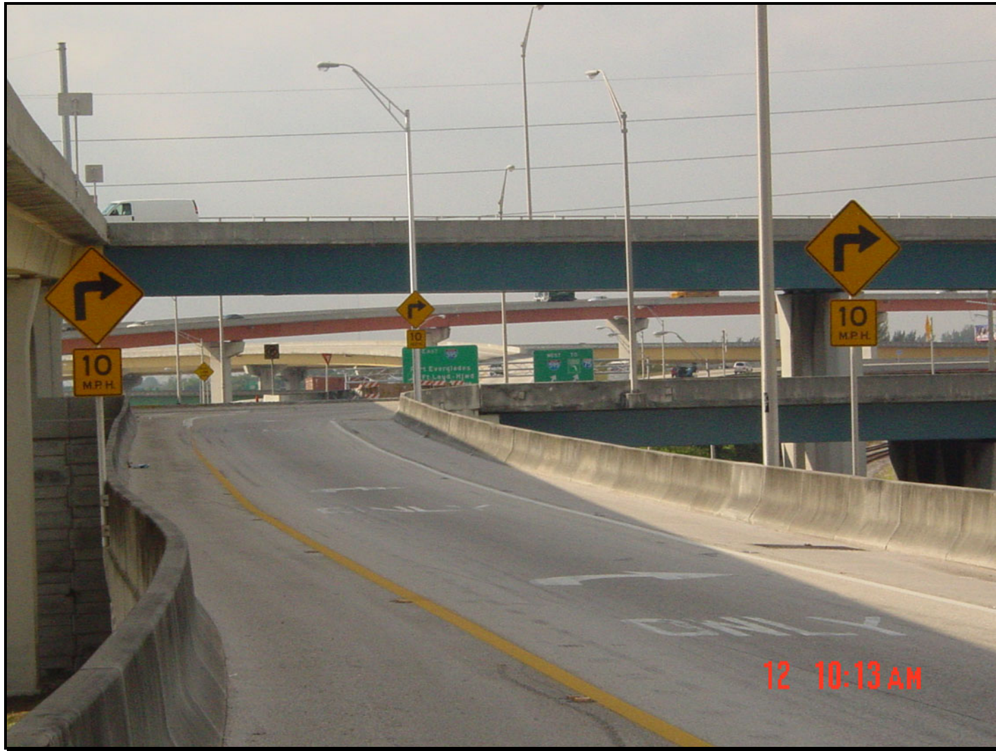
Figure 2. Existing Signing and Pavement Markings along the Ramp Approaching SR 84 (Looking South).
