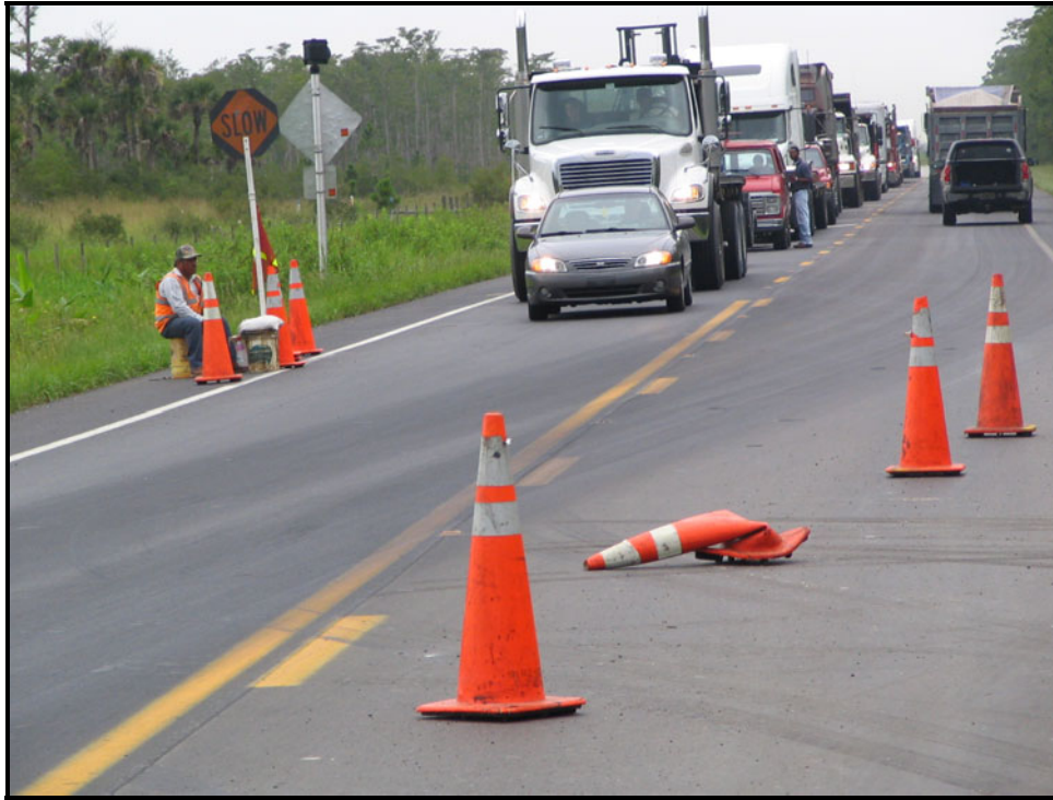
Photograph 5. Typical One-Lane Operation with Flaggers
