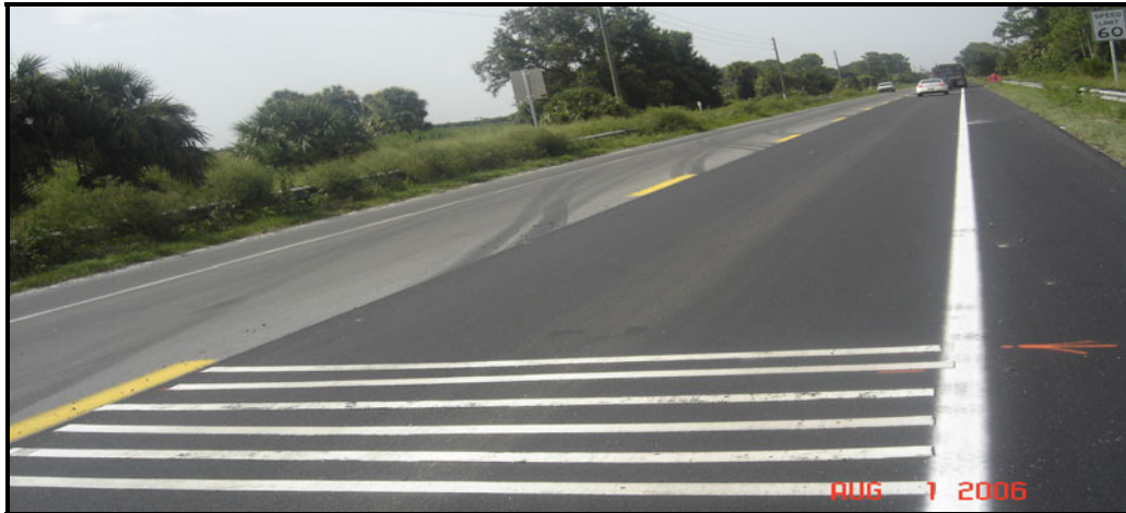
Photograph 4: Typical installation of temporary rumble strips (6 strips per set)
