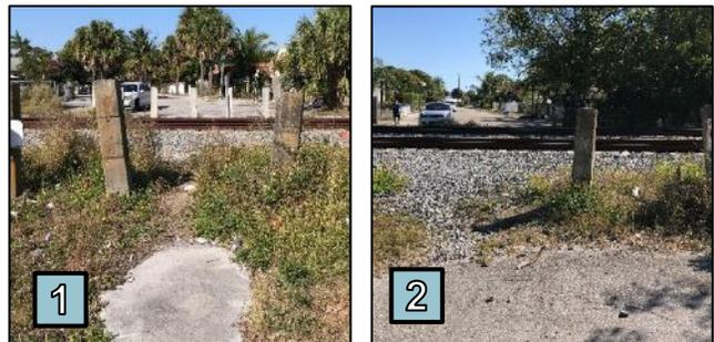
**Recommendation:** Construct **8 ft. hardened fencing** on the east side of the corridor between existing fencing at the ends of El Prado and Ave. Alegre. **Guardrail** is recommended around the cul-de-sacs on the west side. If necessary, **vehicle gates** for FECR personnel should be added on the west side to preserve FECR vehicle access to the corridor.
