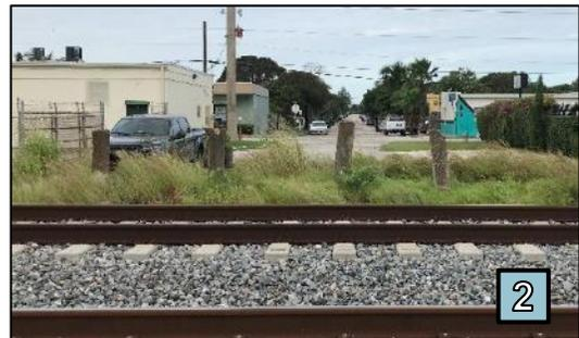
**Recommendation:** Install a **vegetation barrier** along the east side of the corridor between Bunker Rd. and Hunter St. The corridor is open with few barriers to limit access; however, planting vegetation can define the corridor and discourage crossing. Adding **guardrail** is recommended along the right-of-way line to block use of the driveway at Bunker Rd. It is also suggested that any overgrown vegetation be trimmed that might be used to hide loitering within the existing right-of-way.
