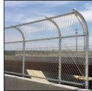
Figure 30: FDOT Standard Bridge Fencing
