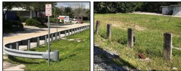
Figure 18: Guardrail and Bollard Barriers
