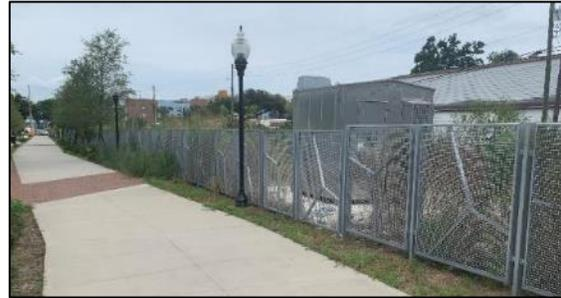
Figure 8: Channelization and Decorative Hardened Fencing on the CFRC
