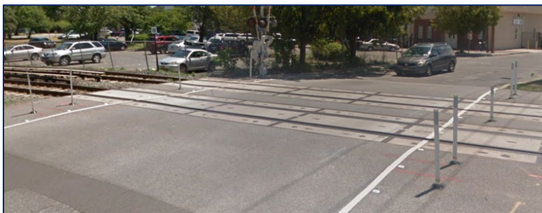
Figure 9: Example image of delineator and edge striping installation at LIRR
